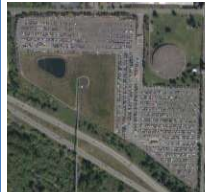
Existing NEPL Facility
