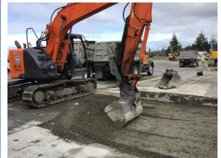
Excavation of distressed individual Portland Cement Concrete Pavement.
