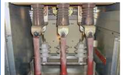
Shown here (before any cleanup) is the interior of switchgear that was protected by SEL, light-sensing and overcurrent protection during a 6.6 kV arc-flash event. Damage was limited to arcing on the cable termination bolts.
