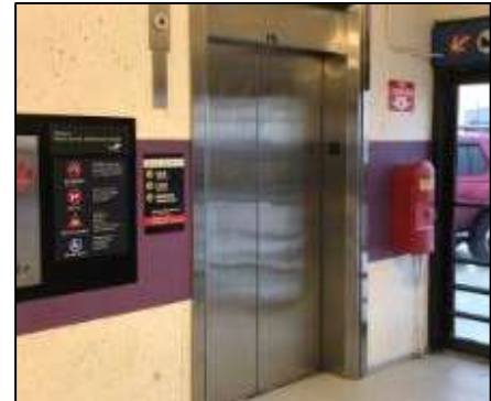
8 th Floor Elevator Lobby
