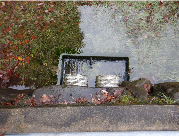
Photograph 1: Catch basin and culverts draining stormwater from the 55-Acre Parcel.
