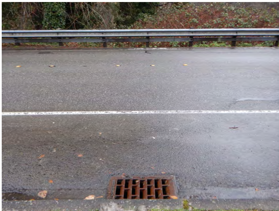
Photo Point 34 Looking North
