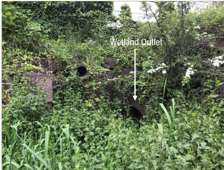
Exhibit 3-5: View of Wetland Outlet, 36-Inch Concrete Pipe, Partially Obscured by Bittersweet Nightshade and Himalayan Blackberry
