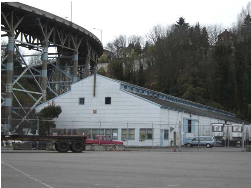
Above, an oblique view of the Northwest Harvest Warehouse, POS Building W-50, east and north facades.
