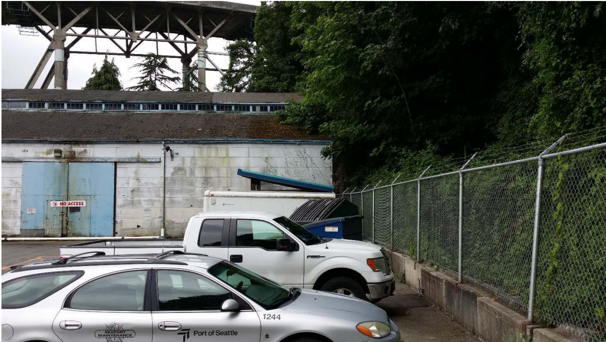
Western edge of Building W-50, with ecology blocks north of the building (looking south).
