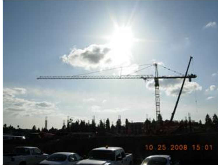
Tower Crane # 1 erected. Looking south
