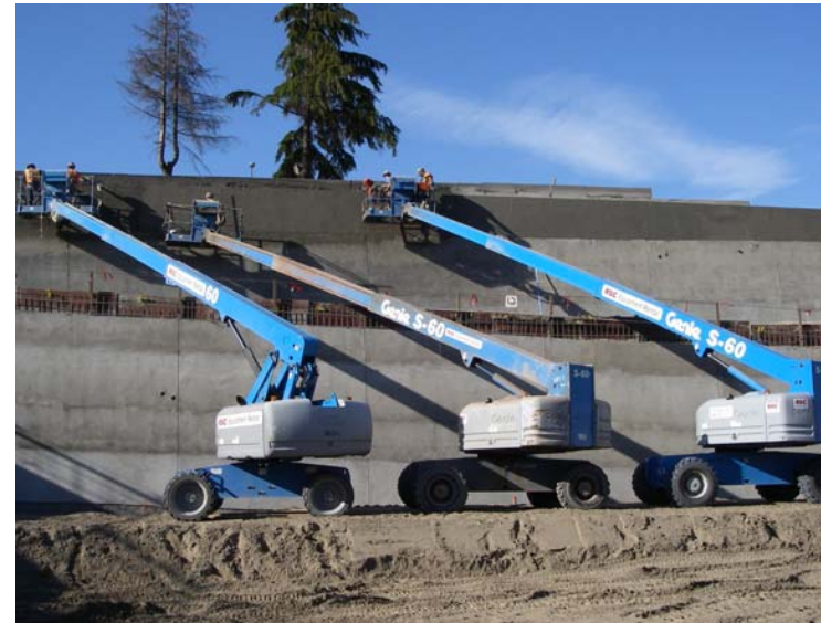
Shotcrete placement was completed on Wall # 1.
