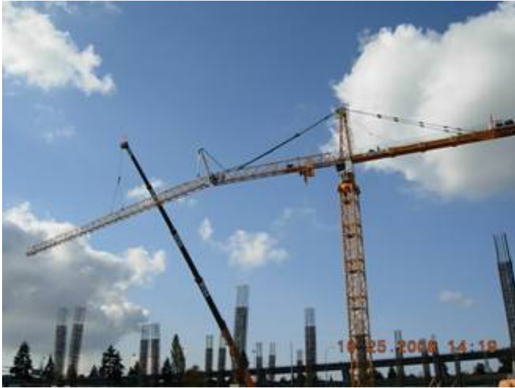
Erecting jib-boom for Tower Crane # 1.
