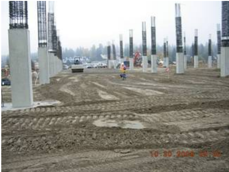
Grading/compacting slab-on-grade in Area A, between columns
