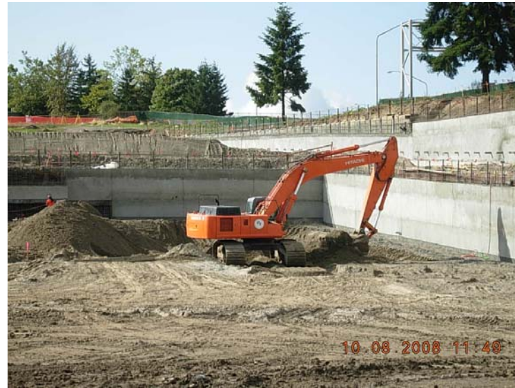
Benching at south end of Wall # 3. Looking west 10.08.2008
