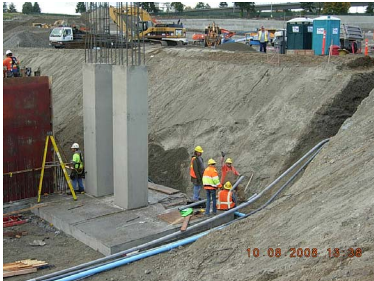
Placing temp. power conduit on N. side of detention vault. 10.08.2008
