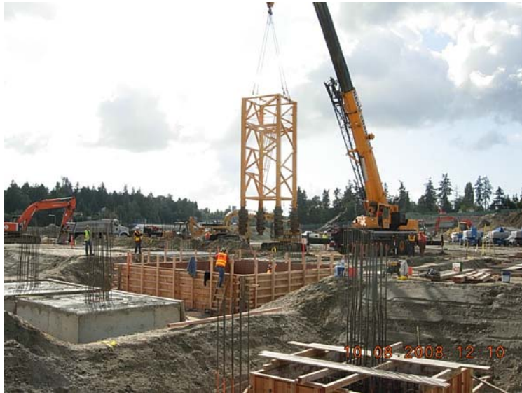
Setting Tower Crane # 1 base in area A. looking SE 10.08.2008
