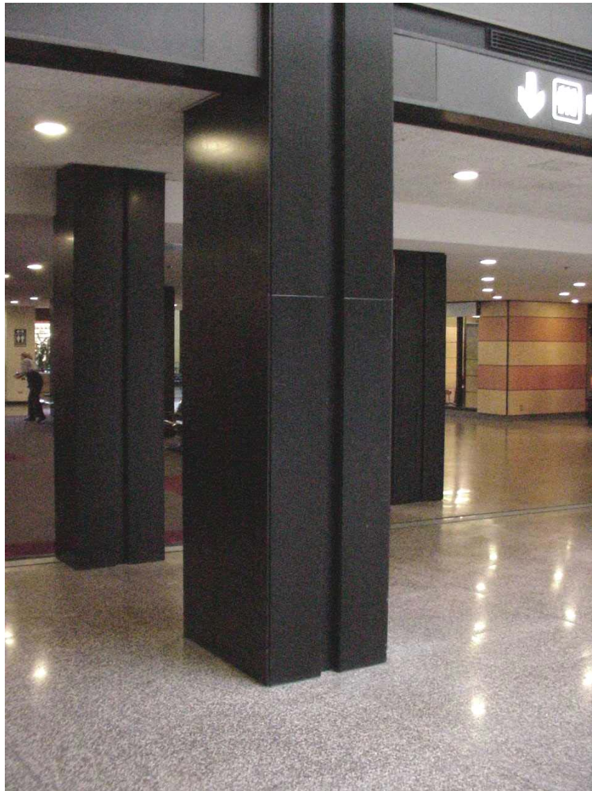
Granite Column Cladding
