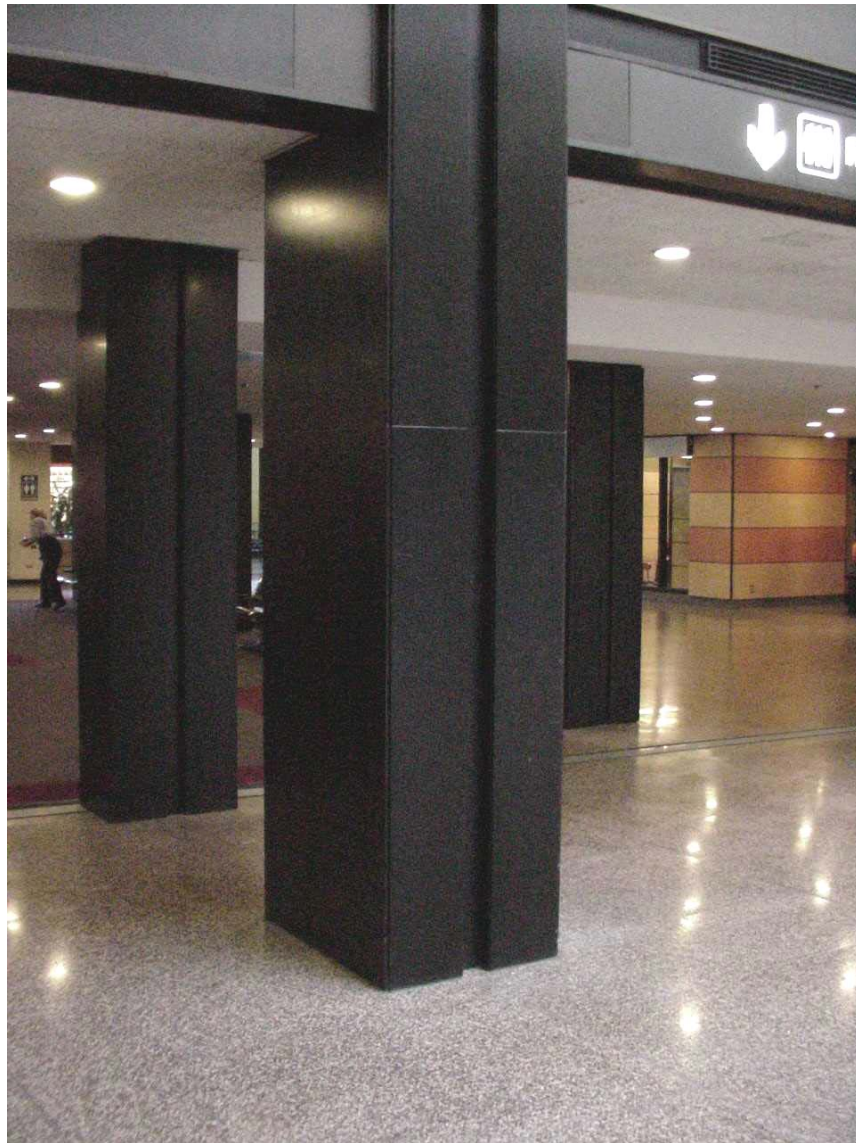
Granite Column Cladding
