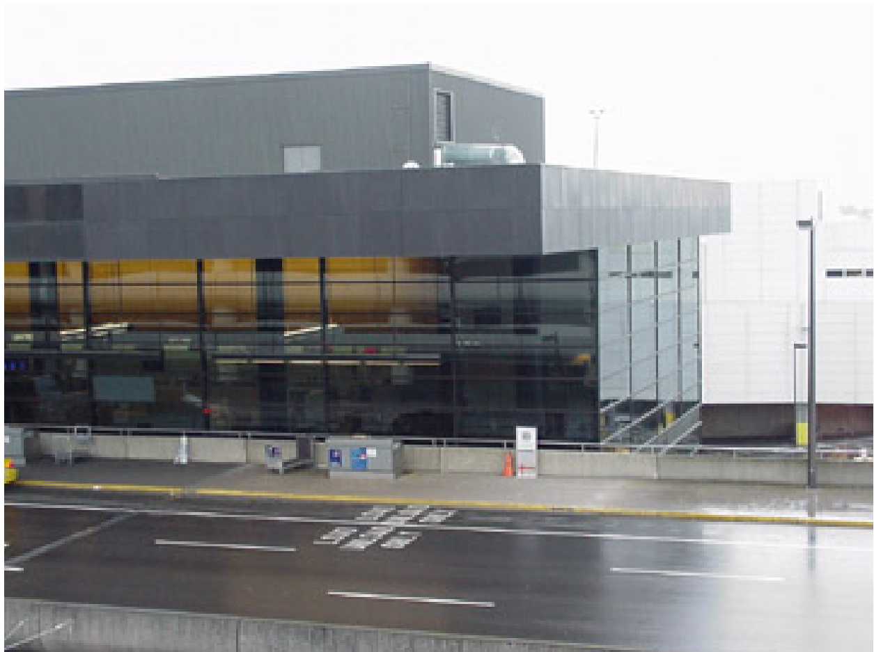
Exterior Metal Wall Panels Main Terminal
