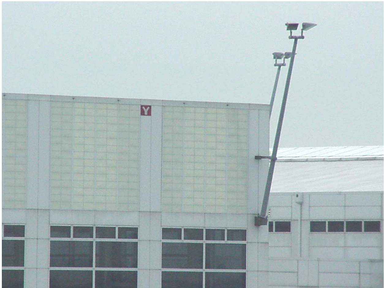
Apron Lighting Poles - Building Mounted
