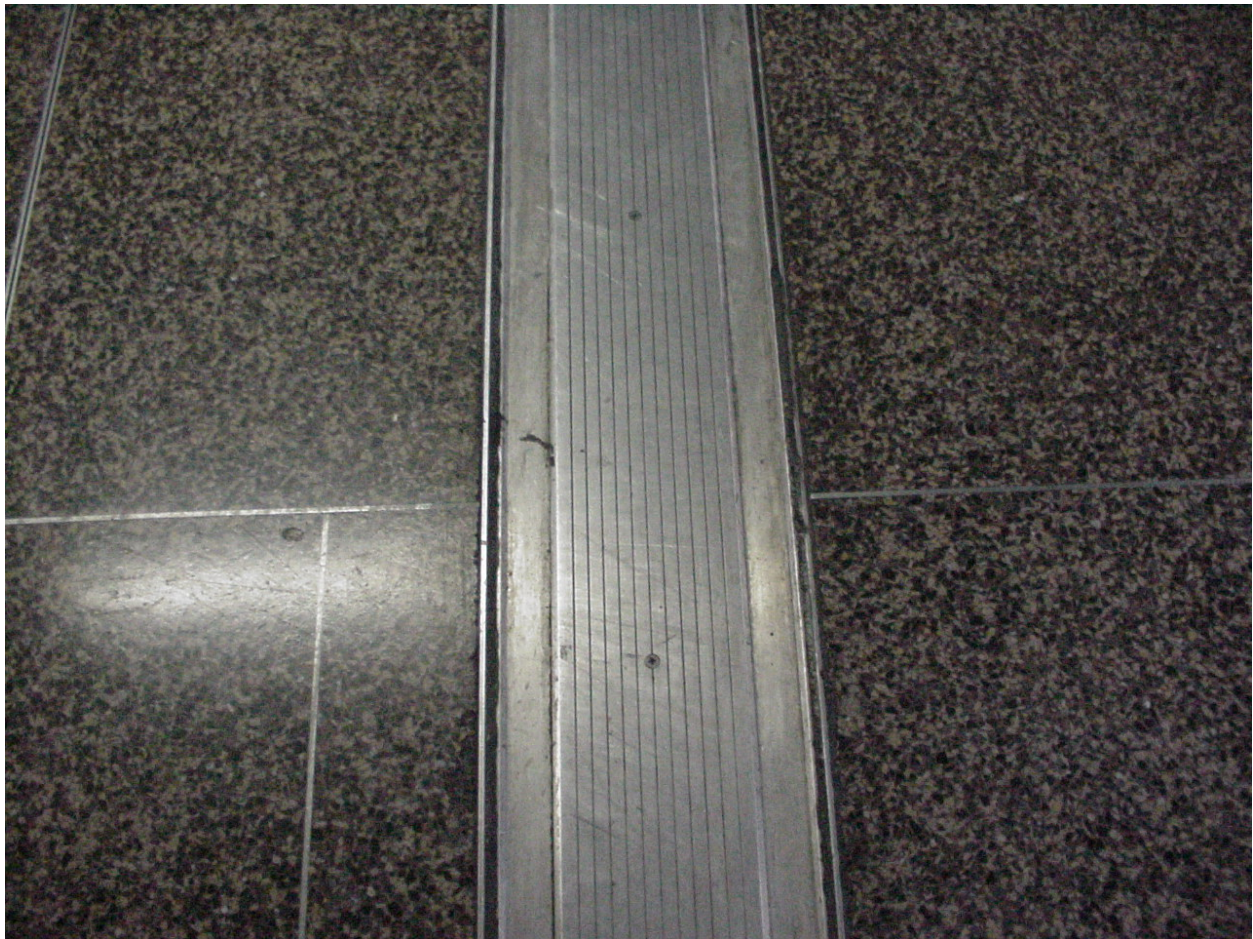
Typical Floor Expansion Joint
