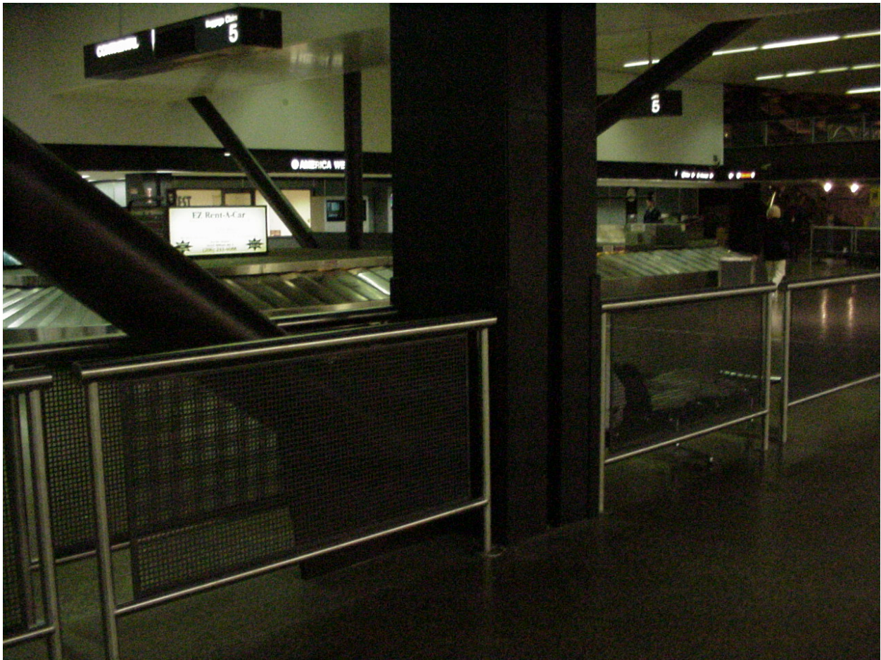
Metal Positive Claim Rail Baggage Claim
