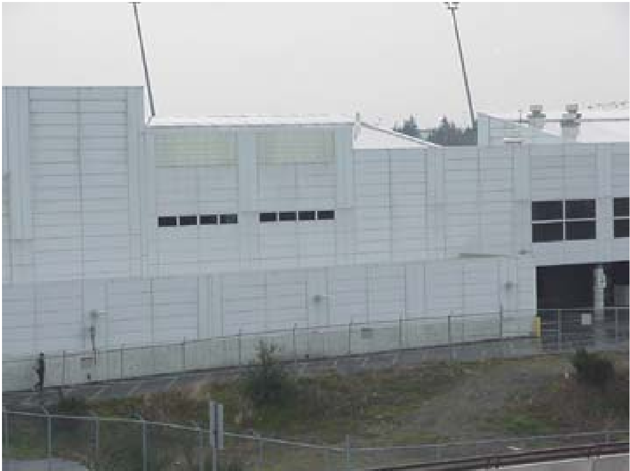
Exterior Metal Wall Panels Concourse D
