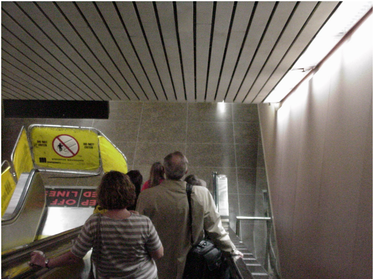
Linear Metal Ceiling Escalator Well
