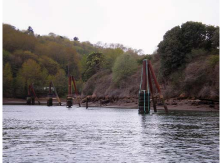
South Kellogg Island, illustrating existing dredged material site, with shoreline vegetation established at upper edge of dredged material deposit. Note barge moorage dolphins in adjacent sub-tidal area (River Mile 1.0)
