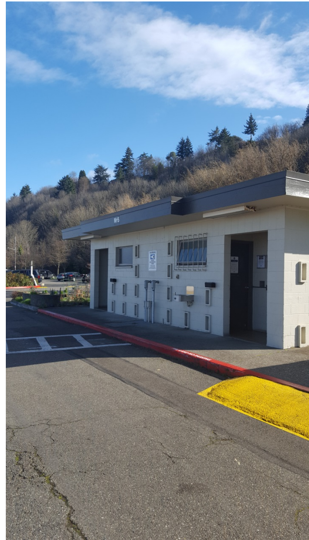
Photo 8 - Building M-5 East Wall Exterior
