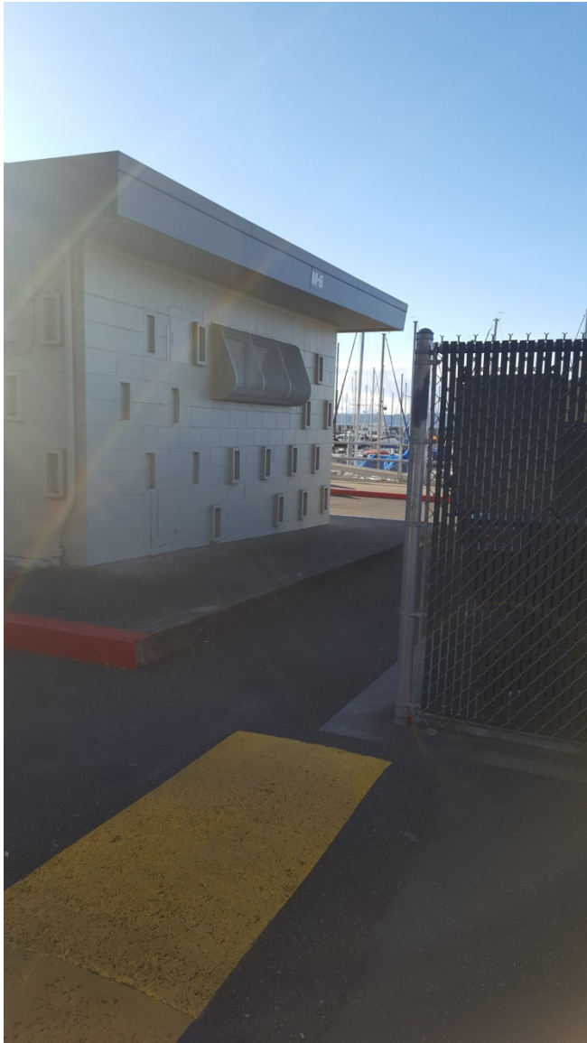
Photo 11 - Building M-6 North Wall Exterior
