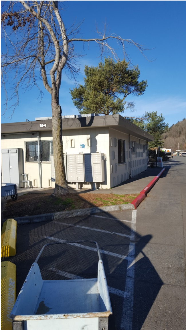
Photo 7 - Building M-4 South Wall Exterior
