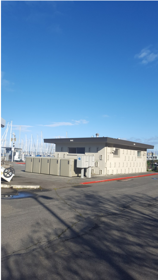
Photo 9 - Building M-5 North and West Wall Exteriors
