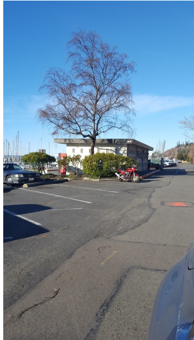
Photo 10 - Building M-6 South Wall Exterior
