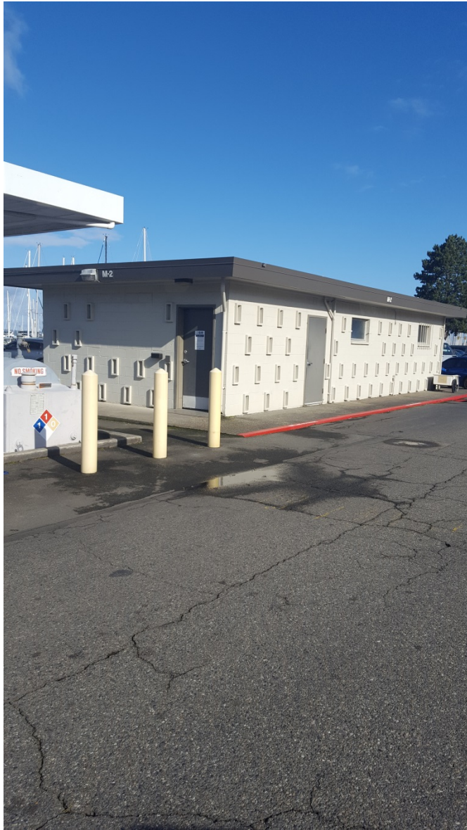
Photo 3 - Building M-2 North and West Wall Exterior
