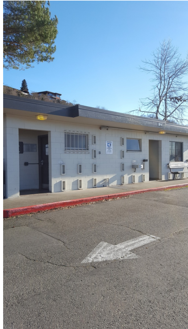
Photo 6 - Building M-4 West Wall Exterior
