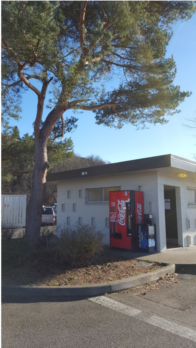
Photo 5 - Building M-4 North Wall Exterior
