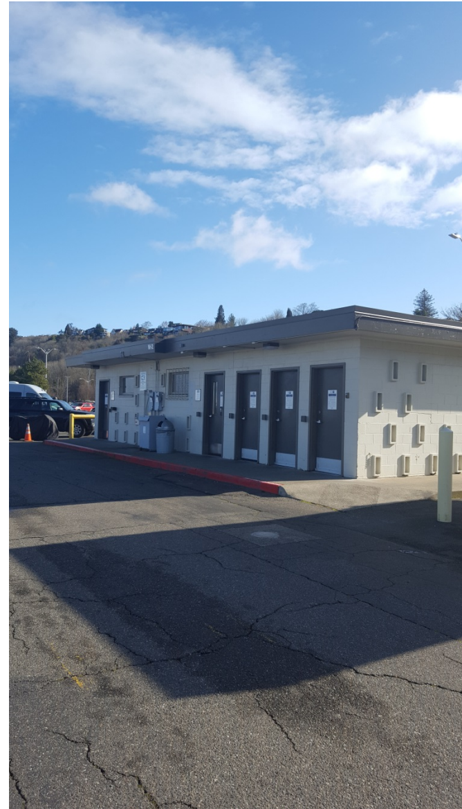
Photo 4 -Building M-2 East Wall Exterior
