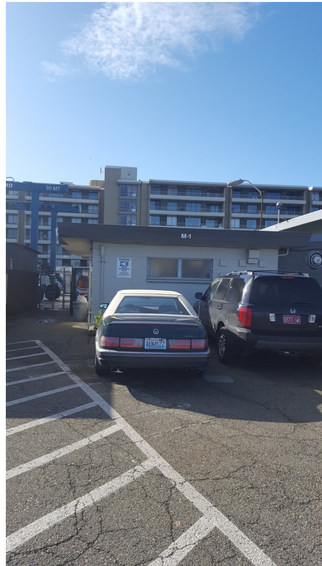
Photo 2 - Building M-1 South Wall Exterior
