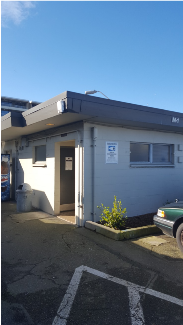
Photo 1 - Building M-1 West Wall Exterior
