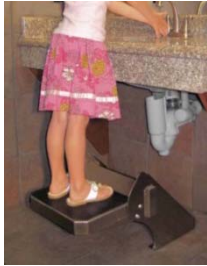
Example child step currently installed in some STIA restrooms
