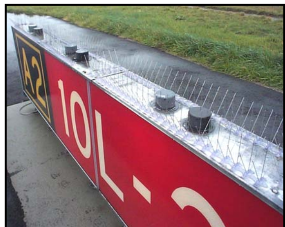
Porcupine wire used to deter raptors from perching near runways (compliments of PDX).
