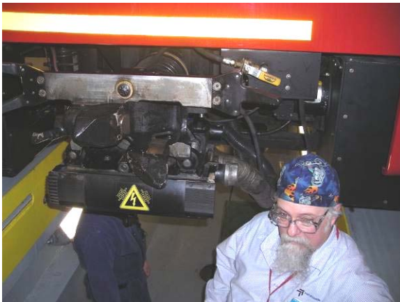
Exiting the shop “pit” under a coupler.
