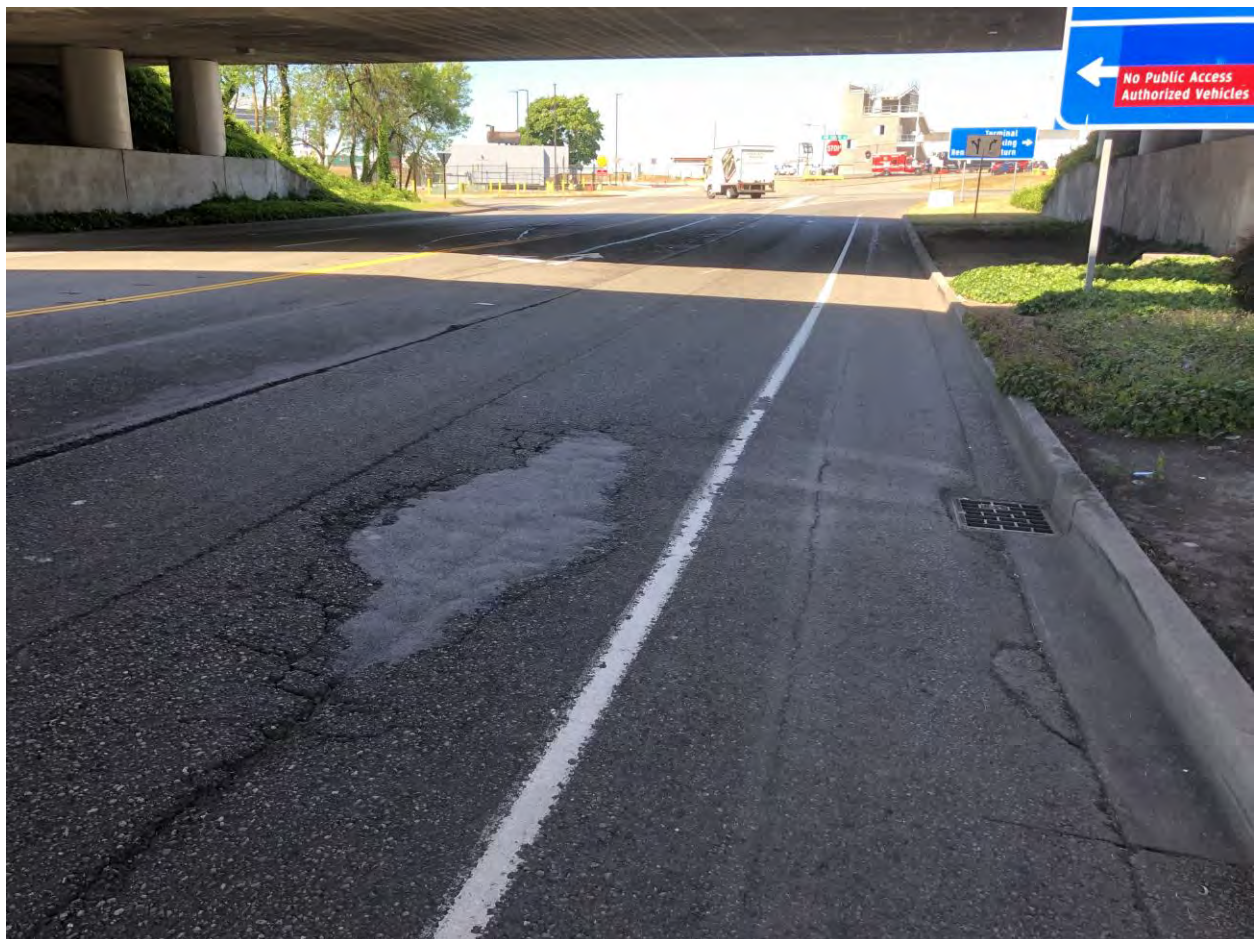
Picture 6. Location of subgrade failure/patching in WB OL (looking west towards intersection with Air Cargo Road).
