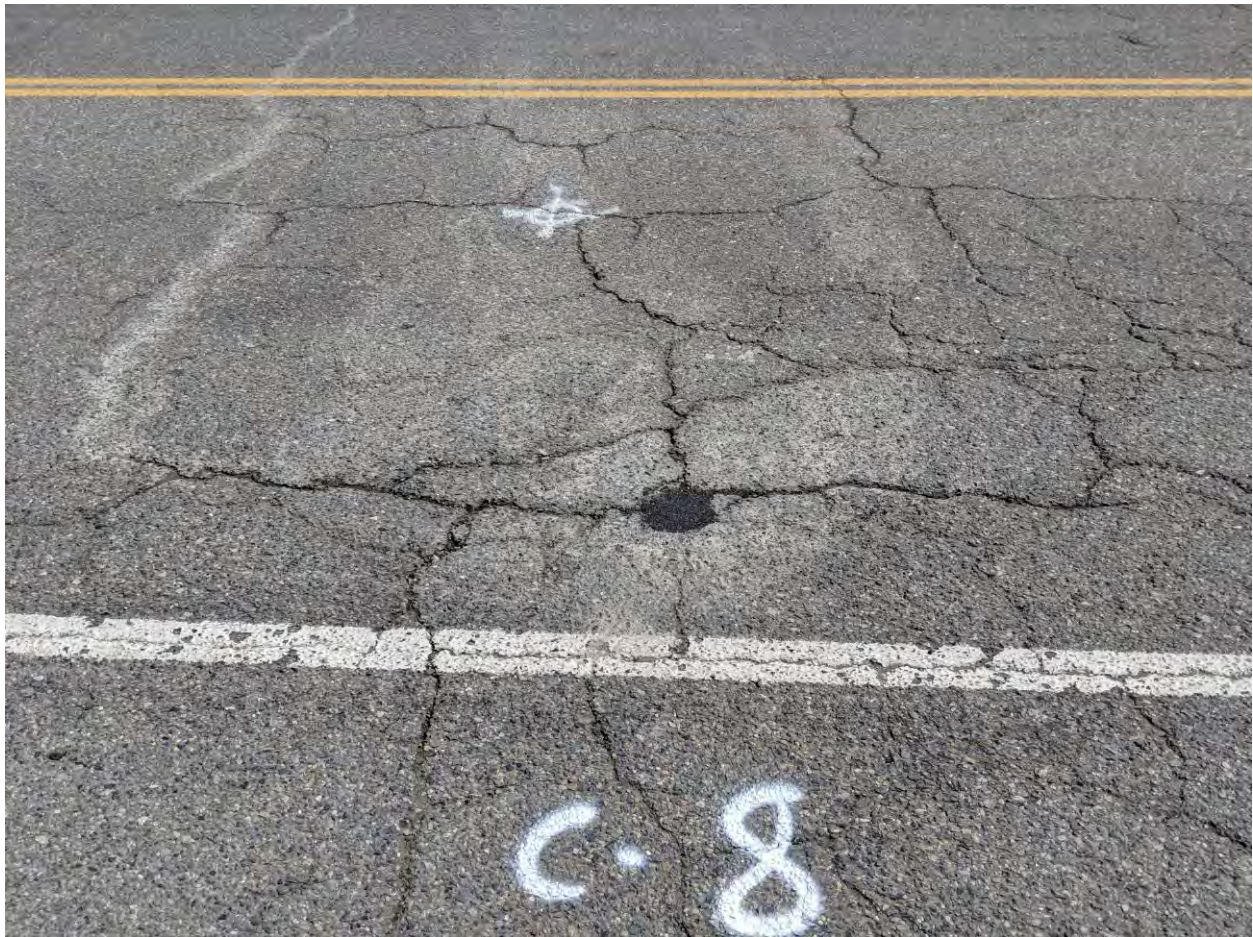
Picture 5. Pavement surface condition at Core-8.
