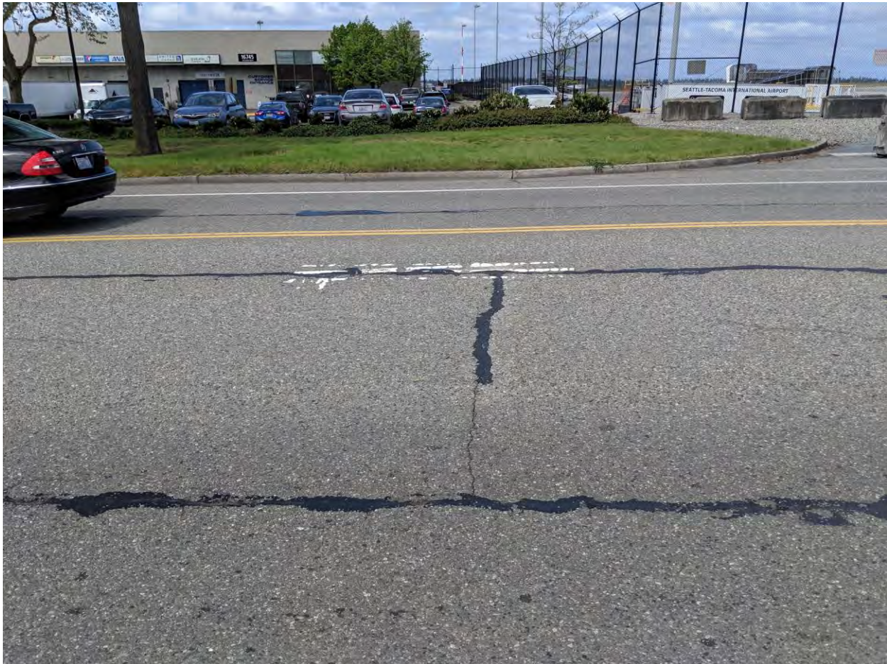
Picture 17. Pavement surface condition at Core-2 (at intersection of sealed longitudinal and transverse cracks in white painted area – looking west).
