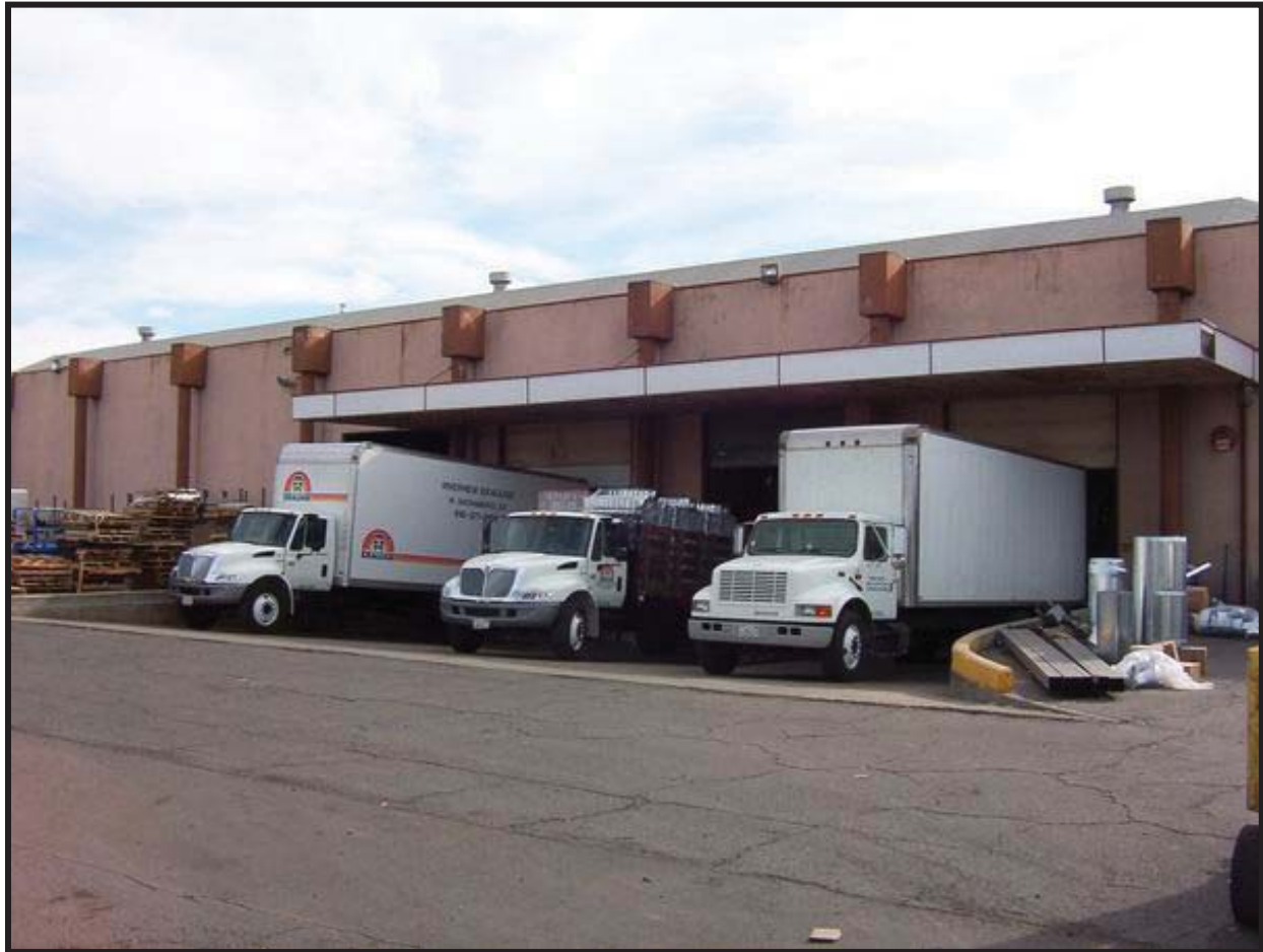
Figure 6. Loading Docks with an Overhang to Prevent Material Contact with Stormwater.
