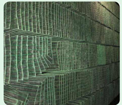
This is a set of MERV 14 filter banks, which filter 90 percent of the particulate from the air.
