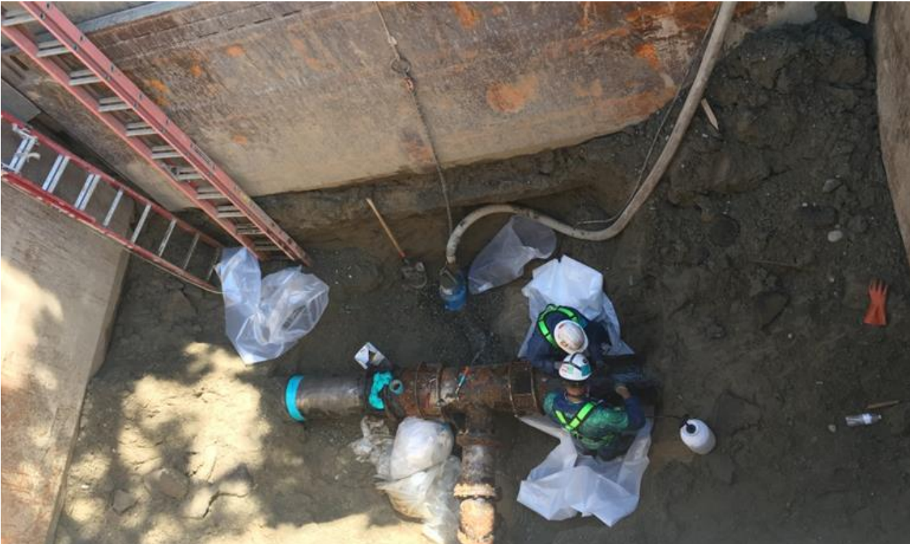
PIPE ABATEMENT – EXPRESSWAY EMERGENCY WATER MAIN REPAIR
