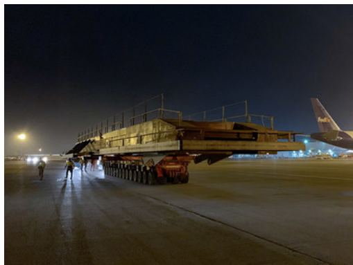
A critical component of the pedestrian walkway (the top chord) was transported during the early morning hours down a closed runway. This same technique will be used to move the center span walkway.
