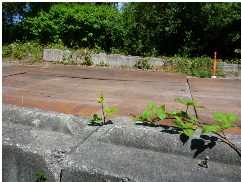
Top: Photo facing upstream (north). Miller Creek draining through the road subgrade, north to south. Buried twin 48" culverts are not evident. Bottom: Photo facing upstream (north). Steel plates cover the damaged road surface over the culverts.
