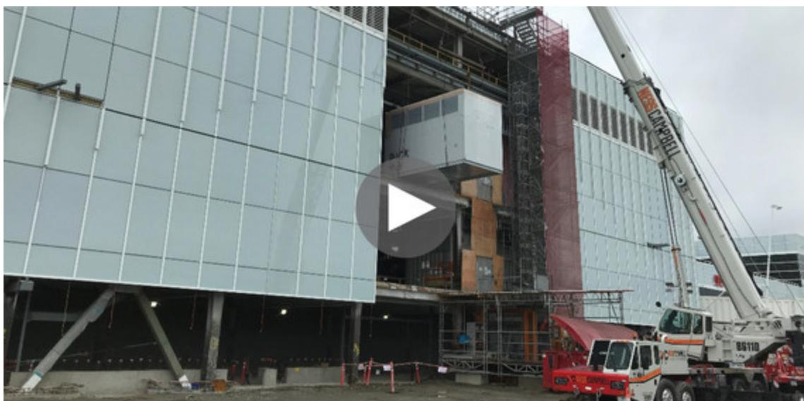
Crews are improving the air quality at the [North Satellite](#) with a new and more robust heating, ventilation, and air conditioning (HVAC) system, a planned upgrade for this modernization project. At the heart of the system are five custom-engineered Air Handling Units (AHUs) built locally in Cheney, Washington. Their massive size required the AHUs to
