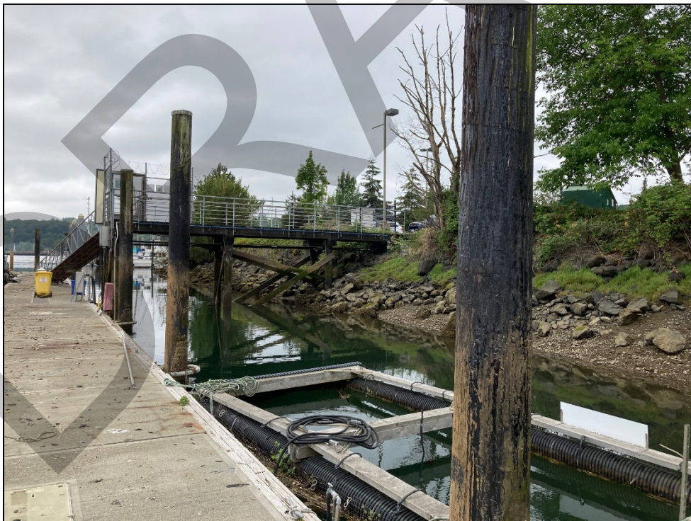
Figure 9. Creosote-treated piles South Float; south pier in background – no work proposed (7/2/21)
