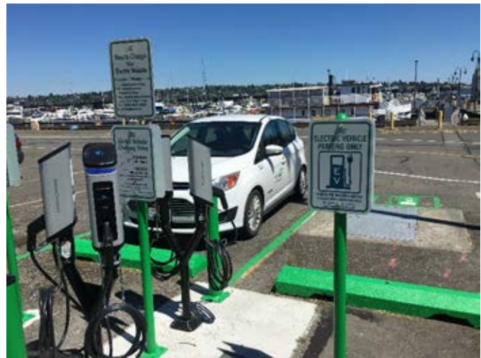
Figure 23. Level 2 EV charging at Fishermen’s Terminal
