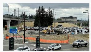
Construction is underway at the cell phone lot, just north of SEA's Main Terminal. Using a segment of the old Airport Expressway, the project will construct a direct access route to the cell phone lot that separates traffic from congestion on S. 170th Street. An improved traffic signal, cell phone lot reconfiguration, and roadway and traffic safety improvements along S. 170th Street and Air Cargo Road are also planned. Learn more $\rightarrow$
