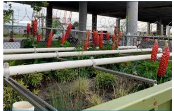
Figure 1. Plants and water distribution pipes at the top of the Horton Street maintenance yard Splash Boxx
