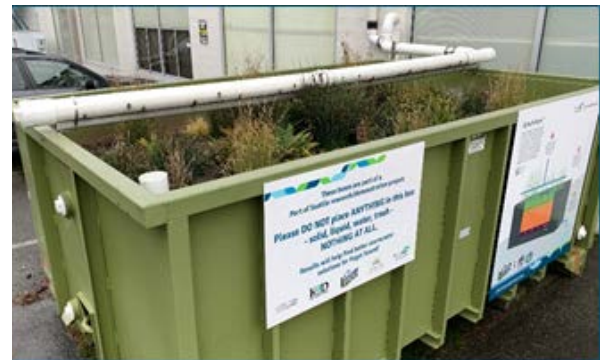
Figure 2. Splash Boxx at MIC receives roof runoff
