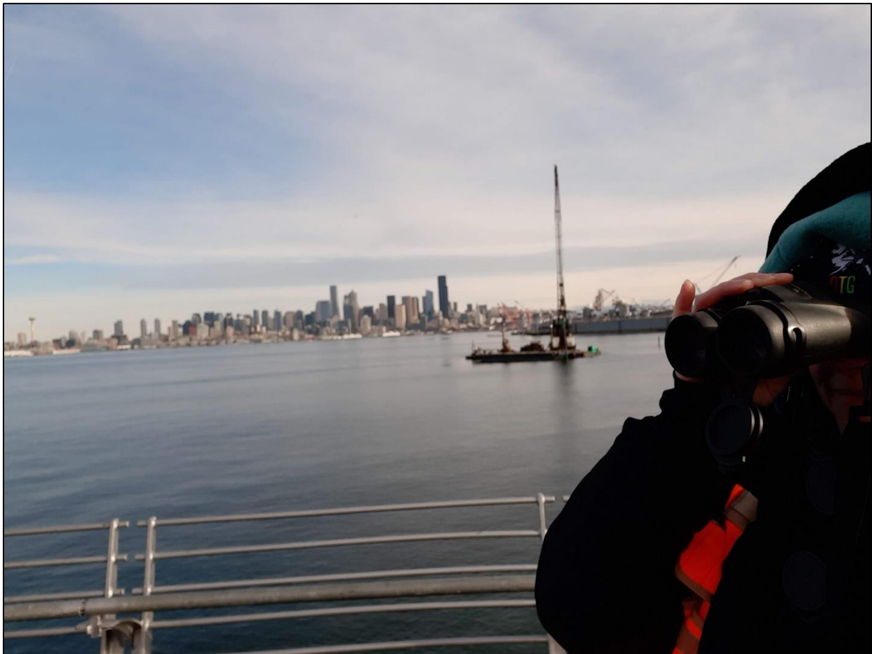
Figure 8. A marine mammal observer watches for protected marine mammals during pile driving operations in Elliott Bay. Credit: Sasha Ertl/Grette Associates
