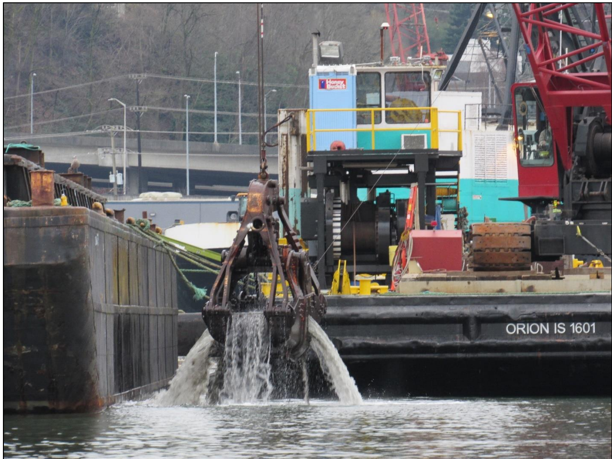
Figure 13. Bucket dredge in use. Credit: Sasha Ertl/Grette Associates
