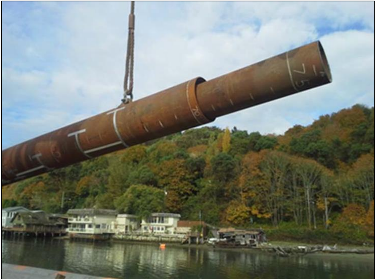
Figure 11. Double-walled pile being suspended above the water in preparation for installation. Credit: Reinhall 2015
