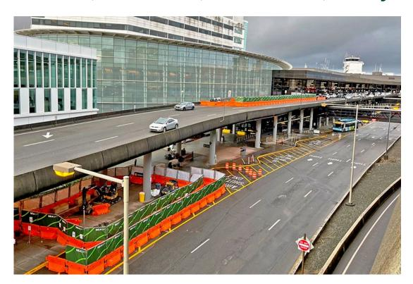
Construction has begun to make SEA more safe, secure, and accessible for all travelers. The curbside accessibility and safety program has begun with construction and installation of bollards (or security posts) along both the Arrivals and Departures Drive curbsides, at the entrances to pedestrian skybridges, and along the courtesy vehicle plaza.
