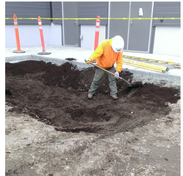
Example soil preparation: subgrade preparation
