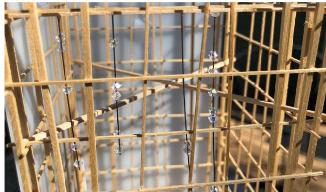
BACK: Prisms on vertical cables connecting at top and bottom to structural tower cross-members.
