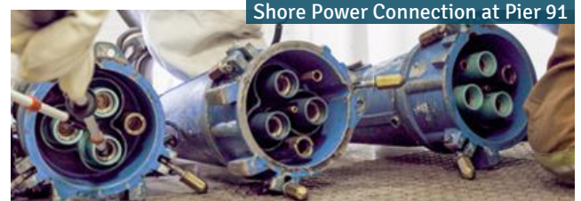
Shore Power Connection at Pier 91
