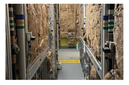
A pipe chase is to be provided behind plumbing walls for access to sinks, toilets, and urinals. These chases also serve as a place to store custodial equipment and supplies, and can be combined with larger custodial closets.
