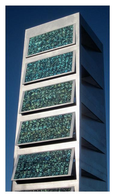
Existing green crystalline photovoltaic panels on the south side of the North Gateway Clock Tower, which may be repurposed when the Clock Tower is removed in the future
