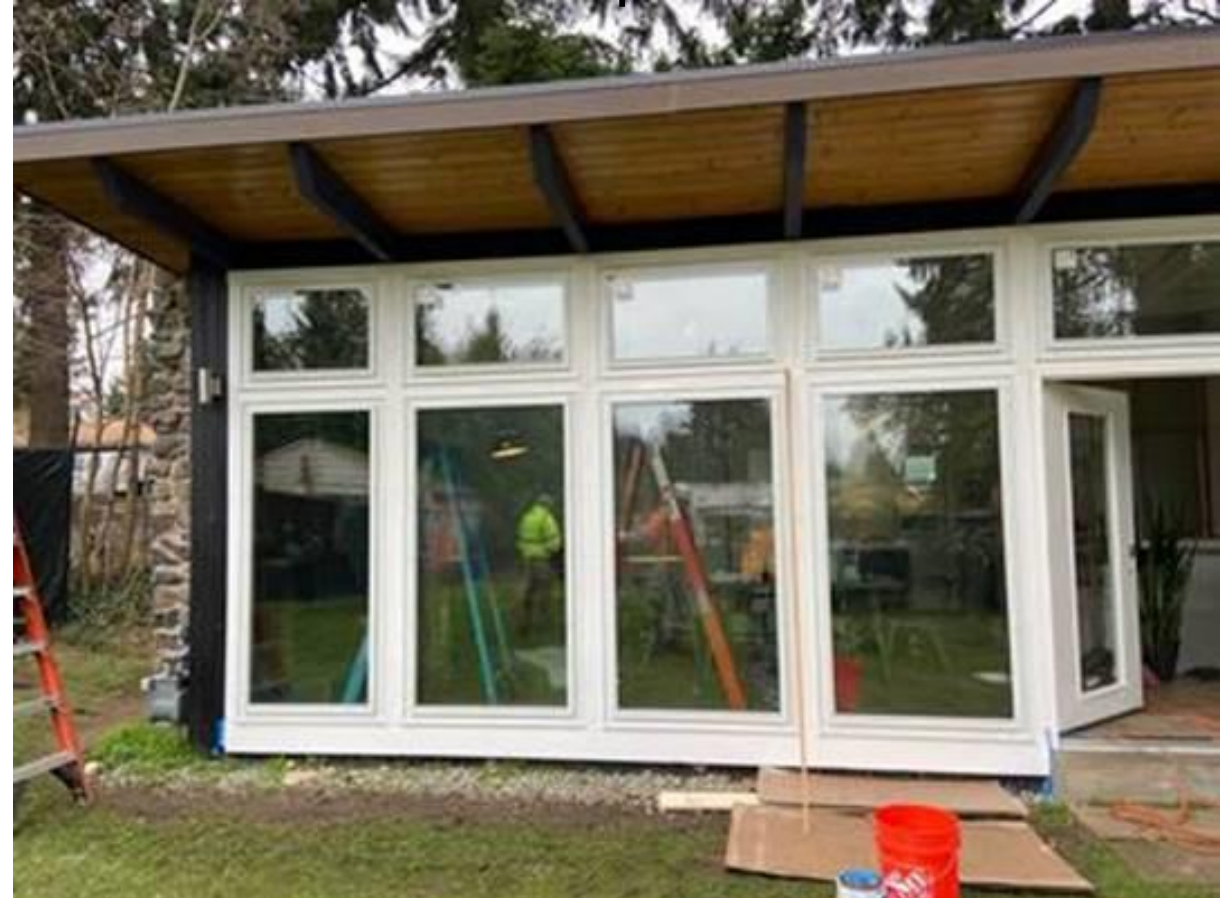
After window replacement
