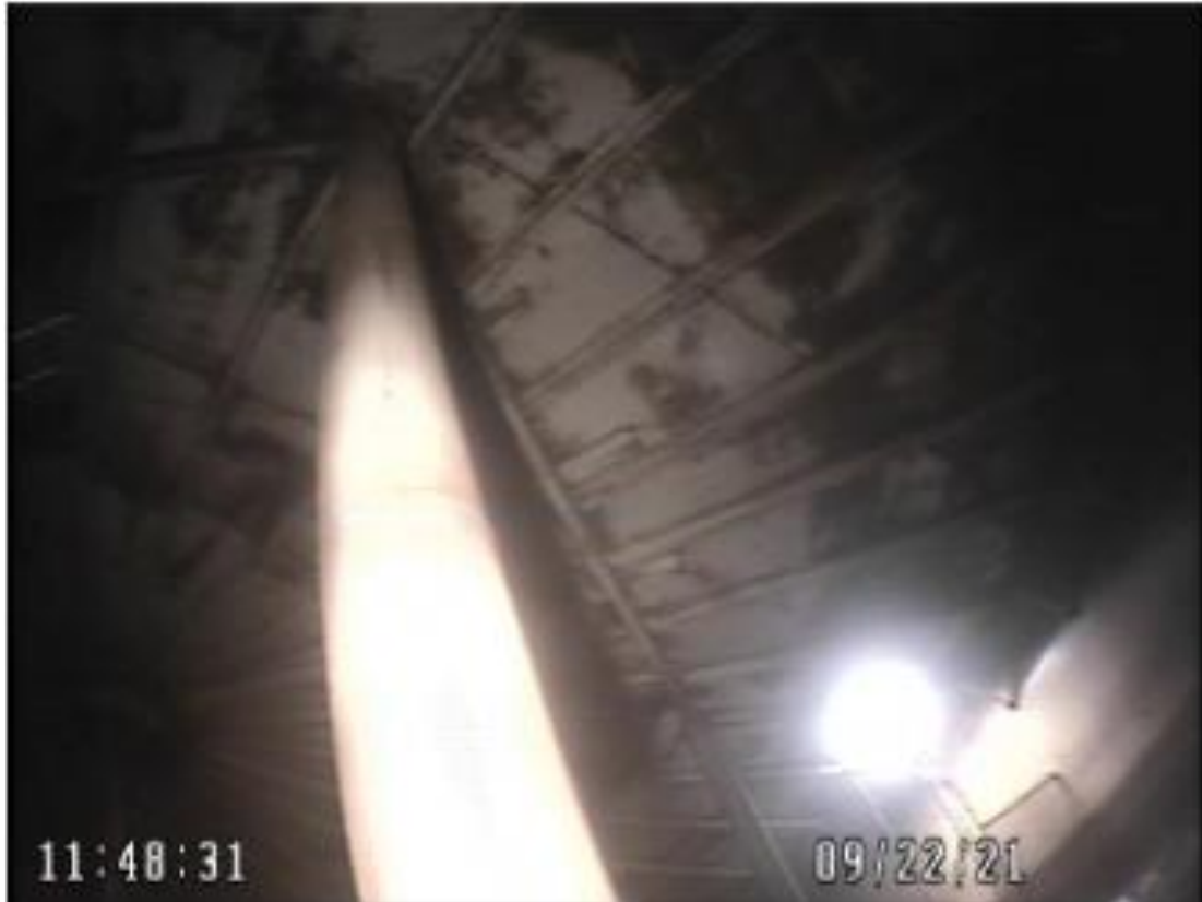
Significant rust on interior tank surfaces
