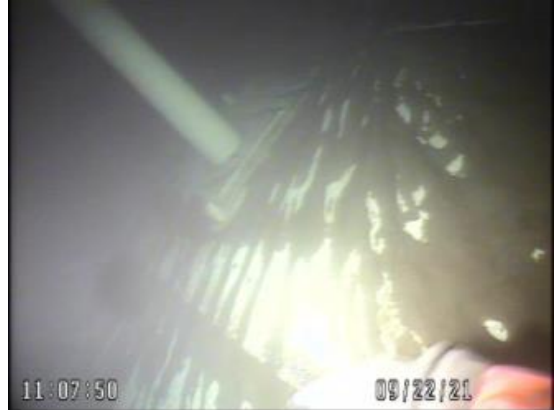
Significant rust on interior tank surfaces
