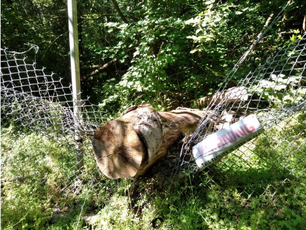
Photo 13: Miller Creek Buffer – Fence line maintenance noted, large tree laying on fence.
