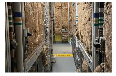
A pipe chase is to be provided behind plumbing walls for access to sinks, toilets, and urinals. These chases also serve as a place to store custodial equipment and supplies, and can be combined with larger custodial closets.
