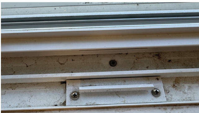
Image of screw installed in sill.
