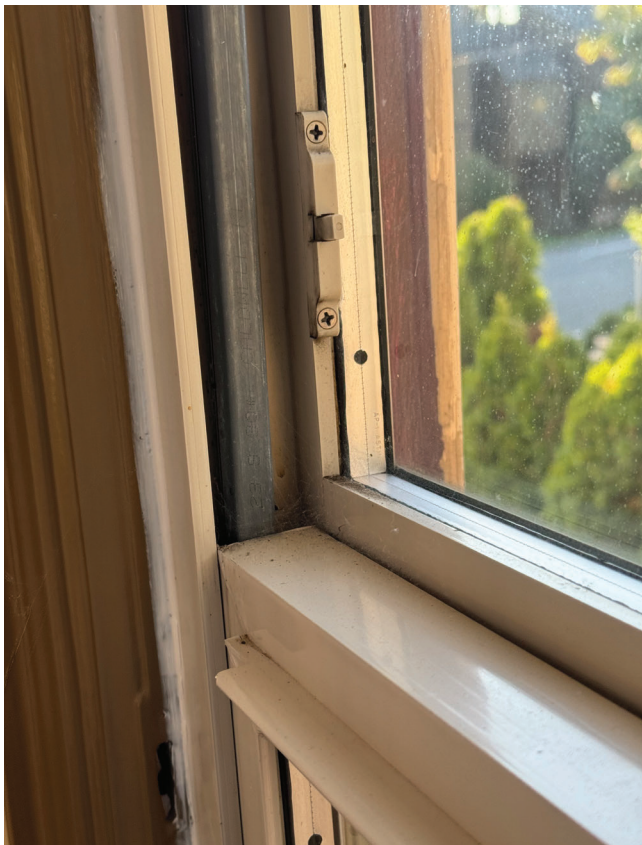
Image of single/double hung window with broken balance.
