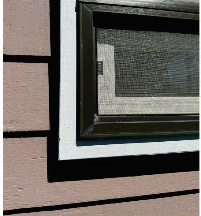
Exterior image of a window and mull covers weephole, as updated install method in and after 1998.
