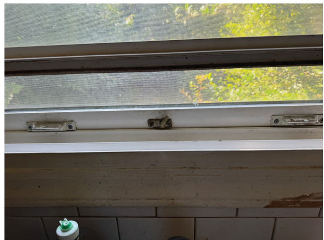
Image of a window with broken/corroded locks.
