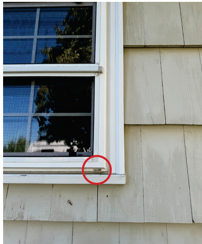
Exterior image of a Milgard window with weephole (circled in red).
