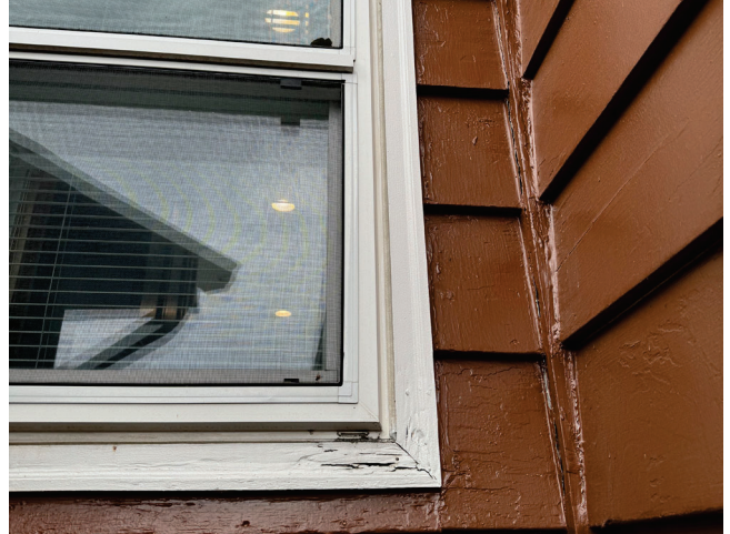
Photo of window trim deterioration.
