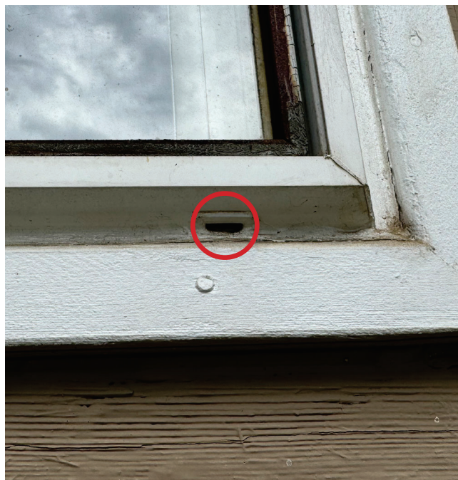
Exterior image of a Alpine (STC44) window with weephole (circled in red).
