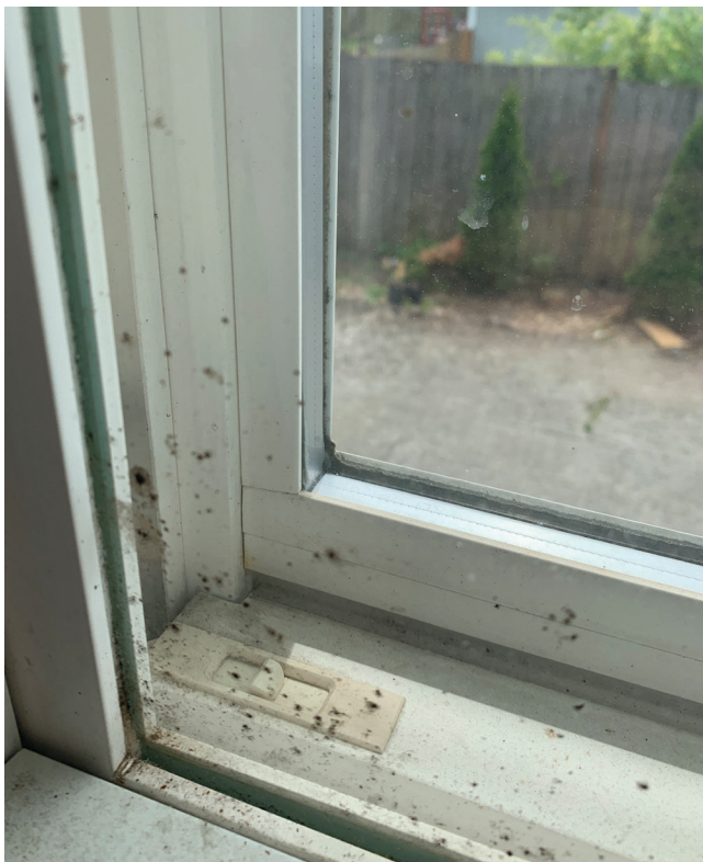
Interior image of a window with possible mold.
