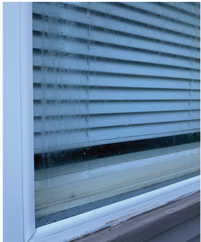
Exterior image of a window with covered weephole and condensation between glass.
