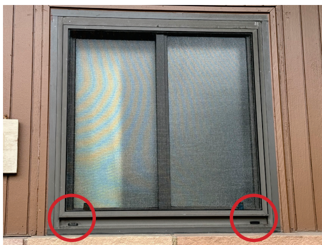
Exterior image of a Peerless/DeVac window with two weepholes (circled in red).
