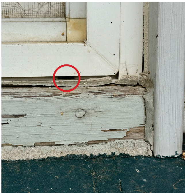
Exterior image of an Alpine (STC44) window with weephole (circled in red) covered by caulking and frame damage.
