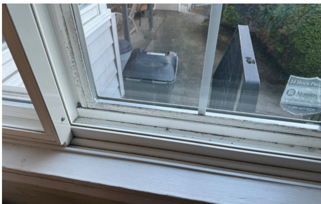
Image of a window with debris between fixed storm windows.
