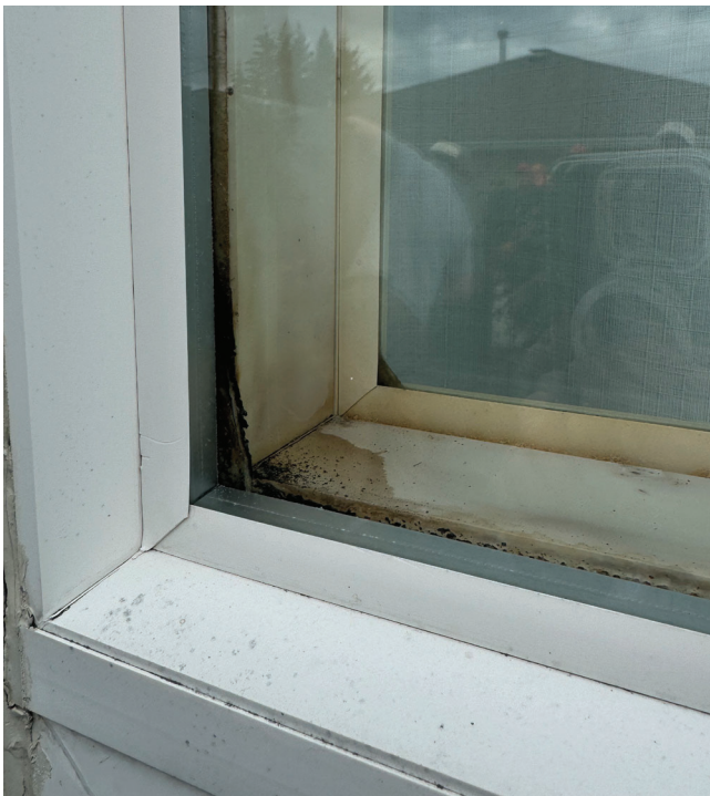
Photo of window deterioration.
