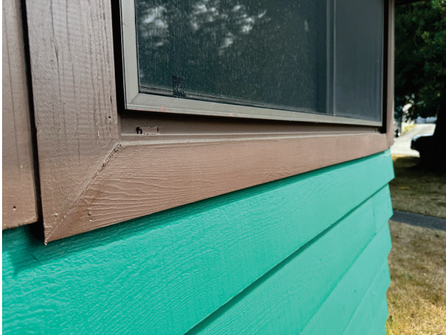
Photo of window with sill painted over.
