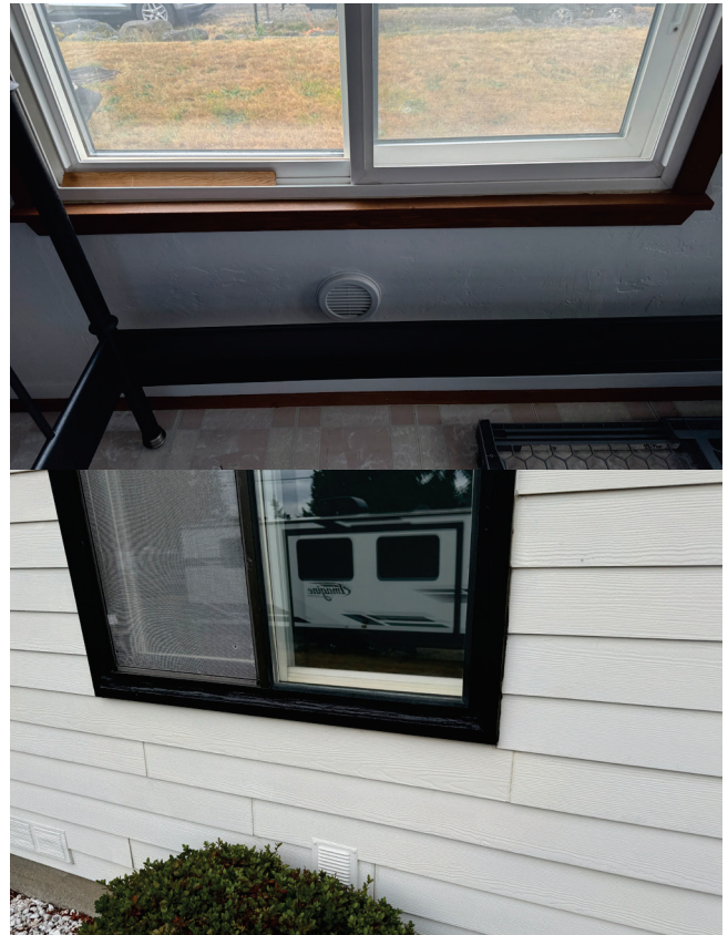
Interior (upper) and exterior (lower) image of fresh air vent path.
