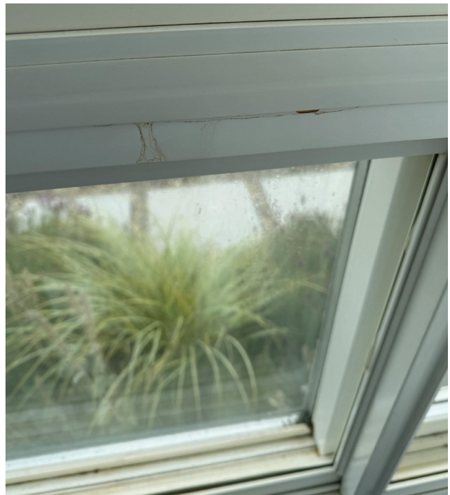
Photo of window with mull leak and trapped debris.
