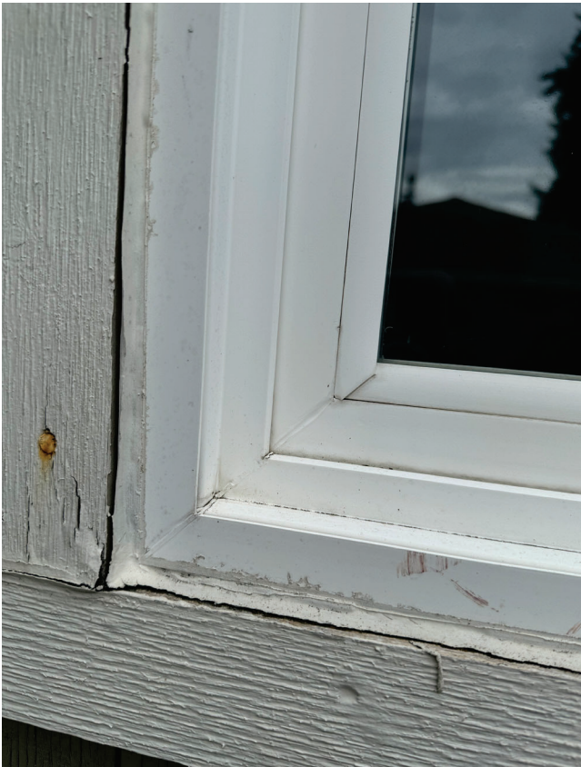
Exterior image of a window with trim damage.
