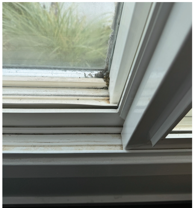
Image of a window with debris between windowpanes.
