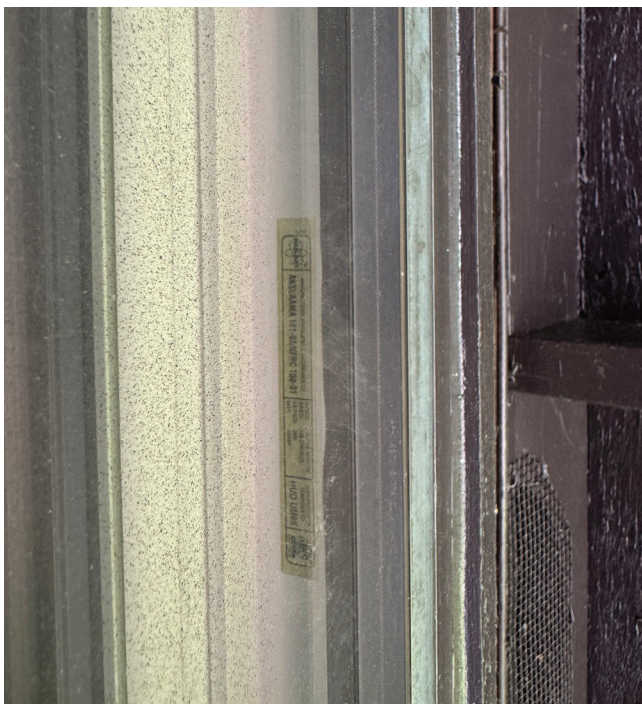
Image of a window with debris between windowpanes.
