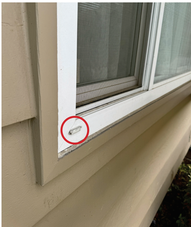
Exterior image of an Alpine (STC35) window with weephole (circled in red).
