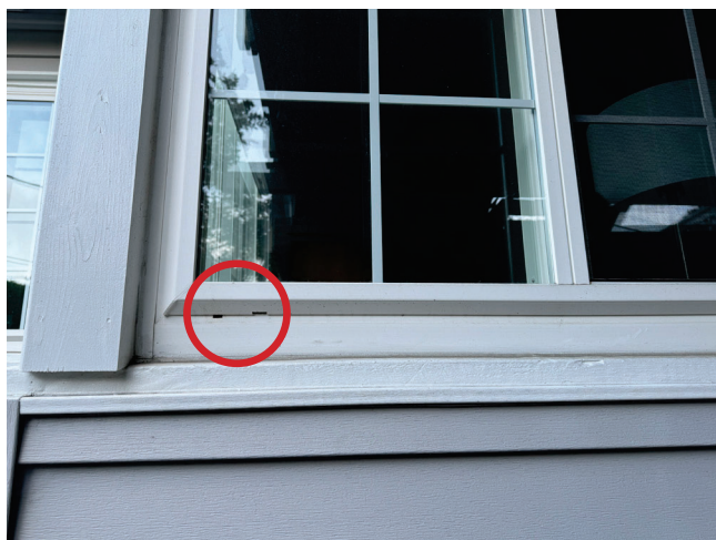
Exterior image of a CDI (STC44) window with dual weephole (circled in red).
