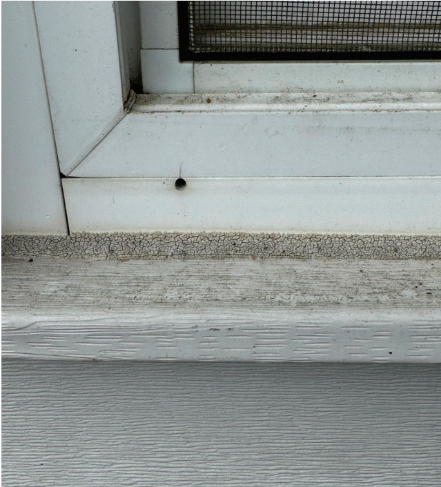
Exterior image of a window with weephole.
