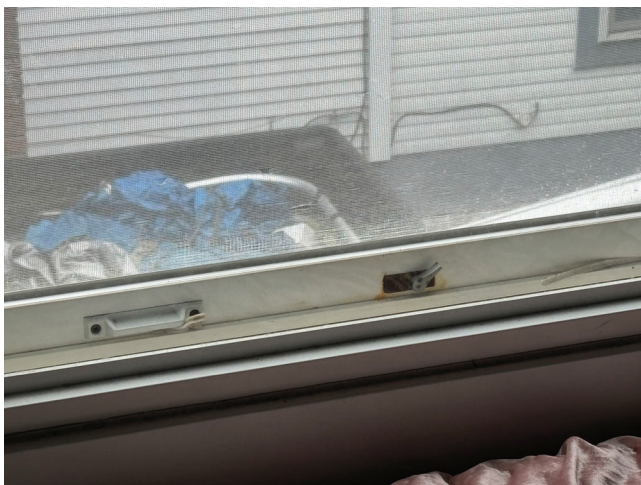
Image of a window with broken/corroded locks.
