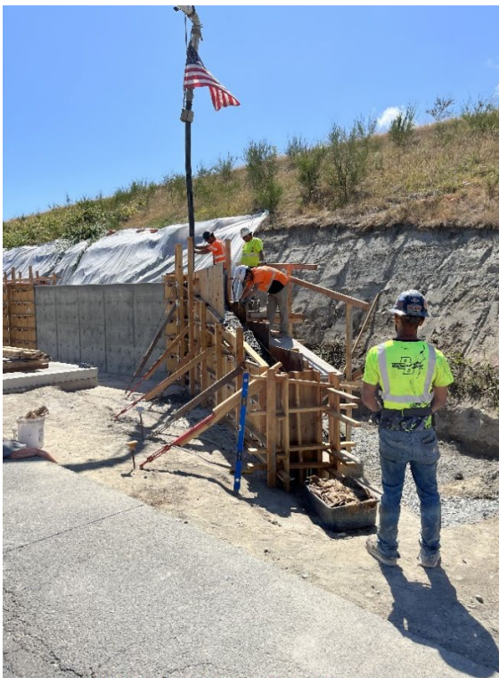
Placing pumped concrete in forms
