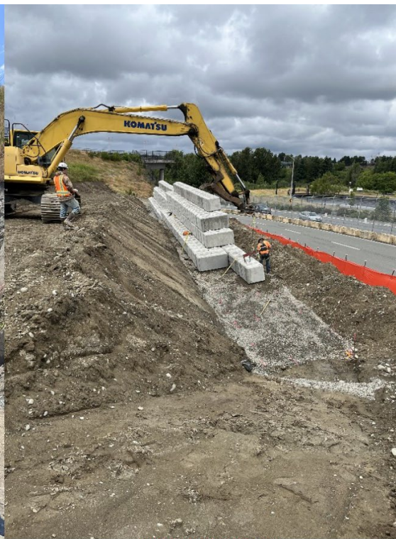
Block wall construction
