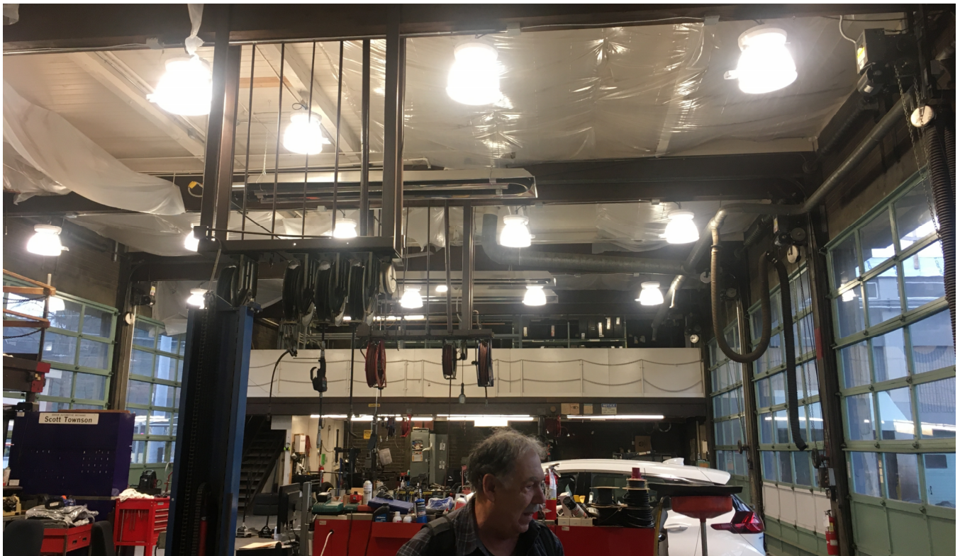
(Lithonia JCBL installed at Seattle Charles Street Tireshop, targeting 50FC, mount height 20 feet)
