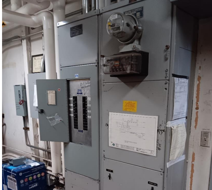
Figure 10: Fisherman's Terminal – Building C-3 Main panel which appears original construction from the 1950s. The age and residential voltage (240/120) of the building are some factors that made this building a lower priority.
