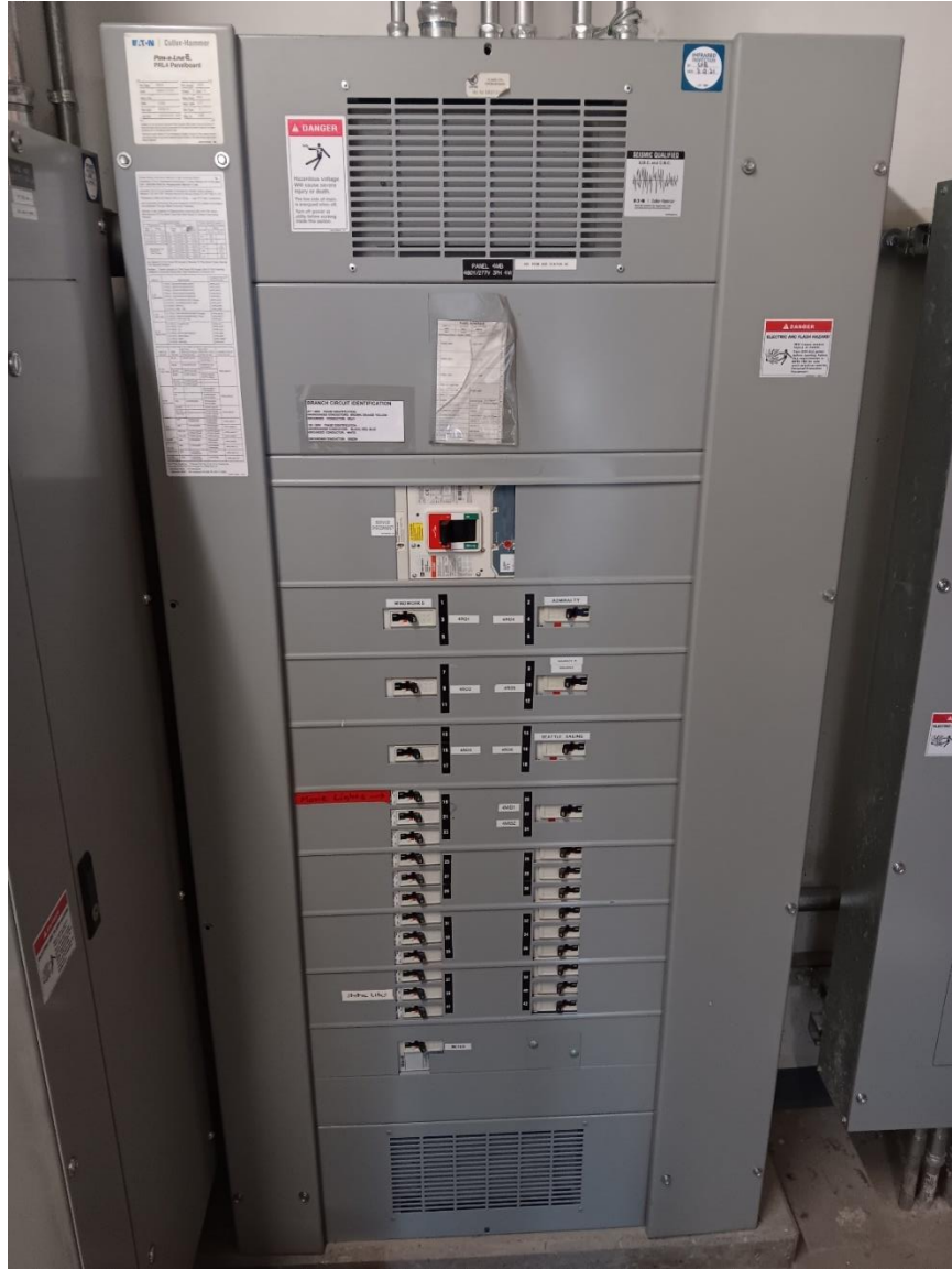
Figure 35: Panel 4MB proposed for interconnection using relocated spares
