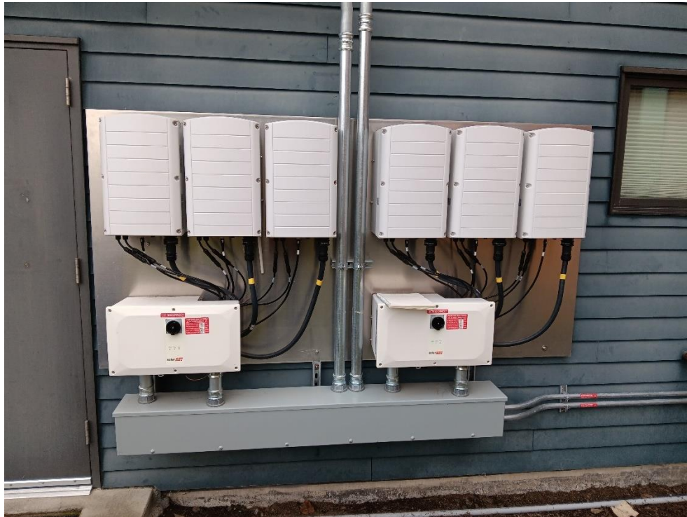
Figure 11: Example showing two SolarEdge inverters mounted to a building wall. This family of inverters was used as basis of design so any Port installations will be standardized across sites
