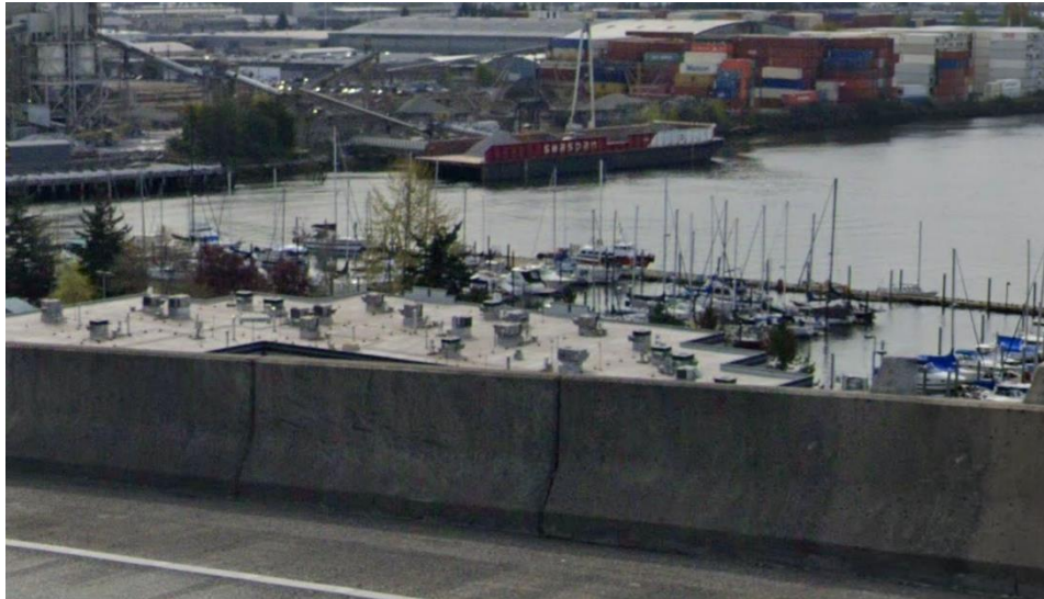
Figure 6: Overhead satellite imagery and Google Street View were both used to evaluate roof complexity and features. This image shows Terminal 102 Building A just above the highway parapet with a complex roof featuring a large number of scattered mechanical rooftop units.
