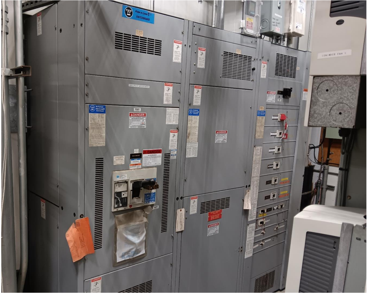
Figure 28: C-175 Main Distribution Panel (MDP). The three breakers expected to be decommissioned are red tagged in the right panel section at the top.
