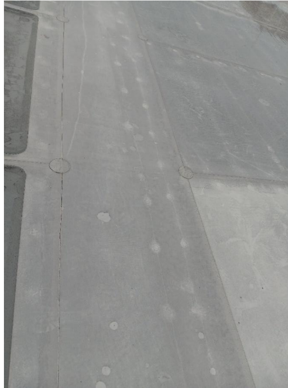
Figure 8: Smith Cove Roof showing wear and discoloration with numerous patches.
