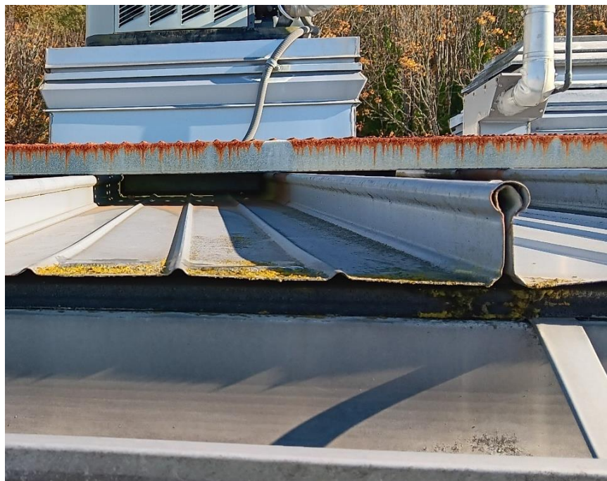
Figure 9: Shilshole A-1 Administrative Building standing seam roof profile. This allows designers to specify attachment hardware for more accurate construction bidding.
