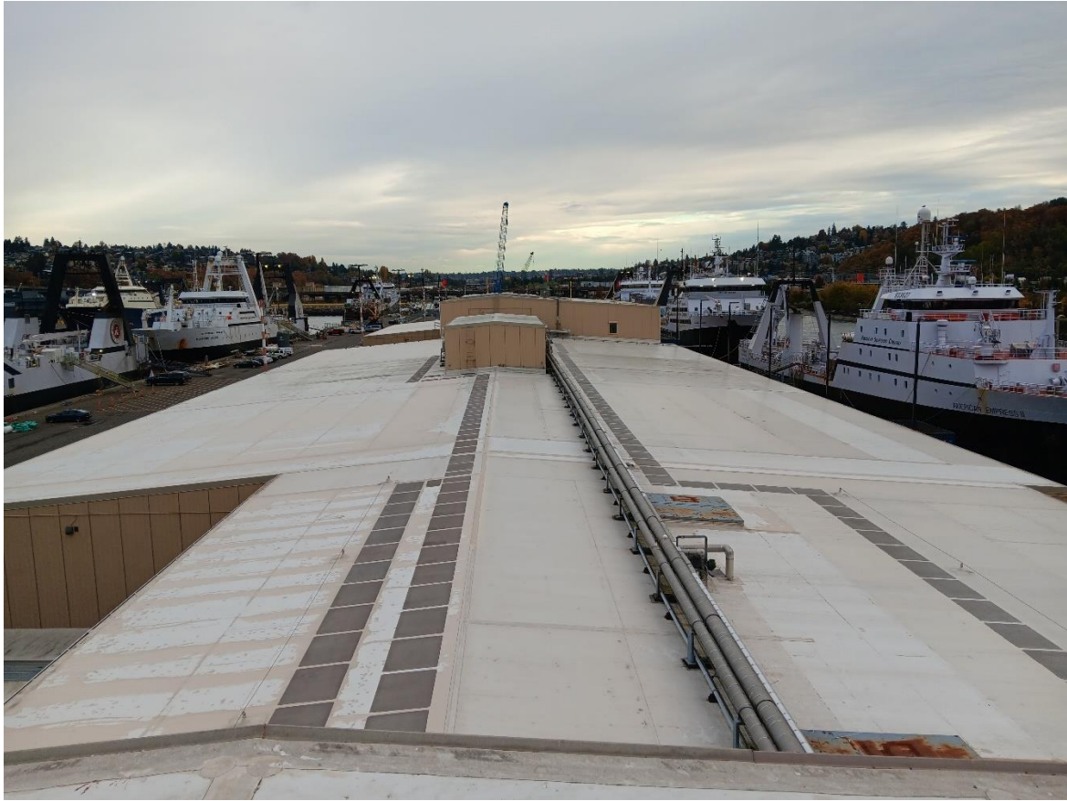
Figure 30: Showing existing roof condition with some minor discoloration, penthouses, and refrigerant lines. Half of the proposed array would be installed immediately south of the small penthouse.
