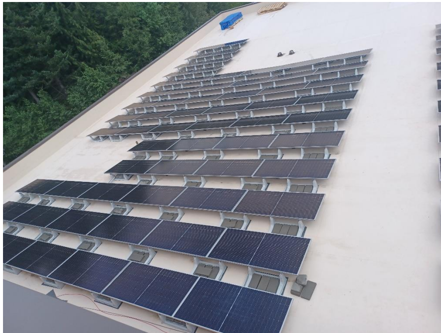
Figure 12: Image shows a ballasted rooftop array like the ones proposed for Smith Cove and C-175. The array is designed around a vent pipe and two drains (top of image) with an access pathway between array sections.
