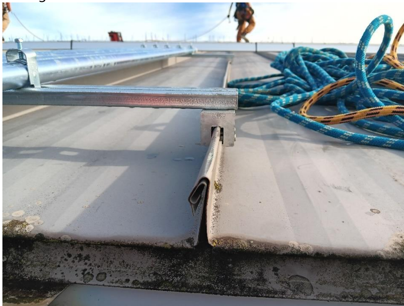
Figure 14: Image shows an example installation on standing seam metal roofing like that proposed for Shilshole A-1. Clamps on the metal roof allow the array to be attached without requiring penetrations to the roof, limiting the risk of voiding the roof warranty.
