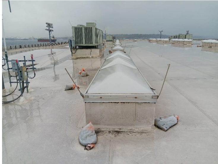
Figure 13: Smith Cove roof showing rooftop air handlers and skylights accommodated with access pathways and maintenance clearances to comply with Fire Code.
