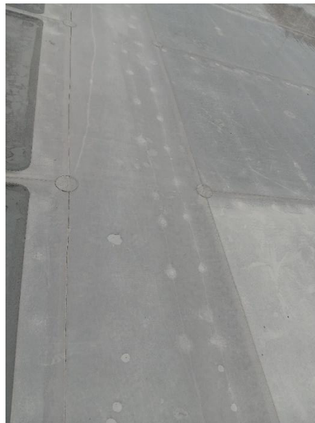
Figure 22: Smith Cove Roof showing wear and discoloration with numerous patches.
