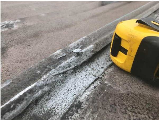
Photo 3: Fastener backout/Split
