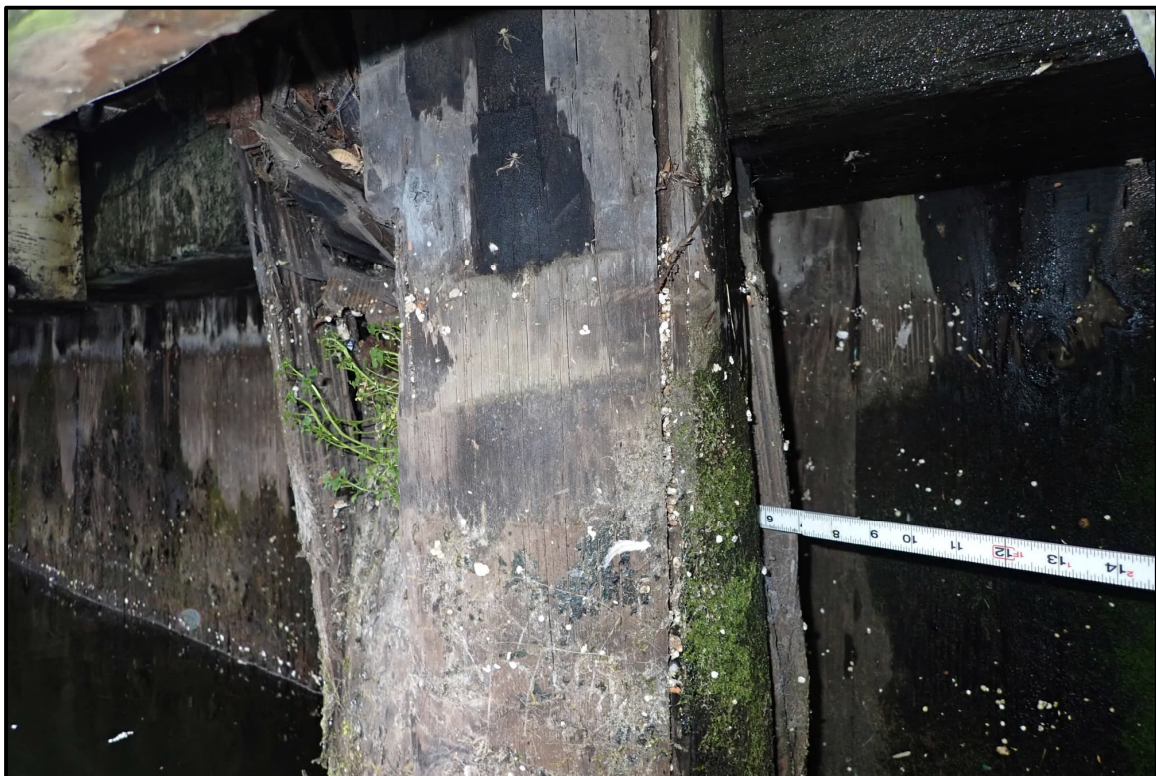
Photo 3-8: Timber pile with severe section loss and splitting at top of pile due to fungal rot along timber bulkhead.
