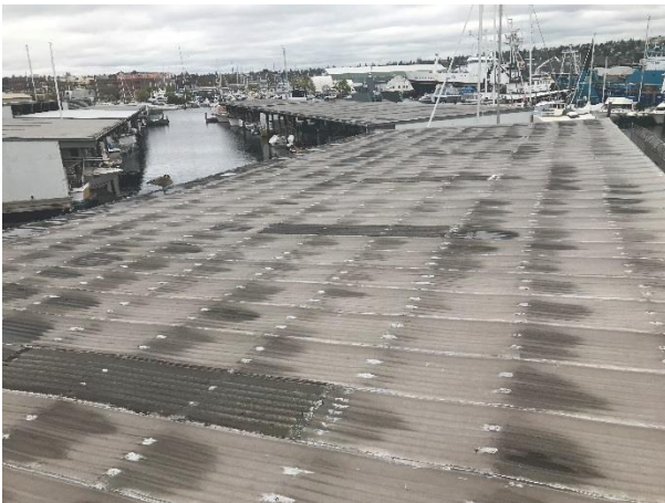
Photo 1: Sealant at EVERY fastener
