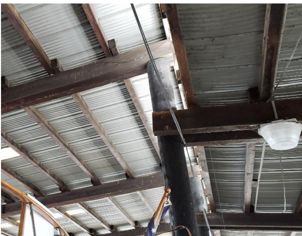
Photo 8: No visible connection at column/beam
