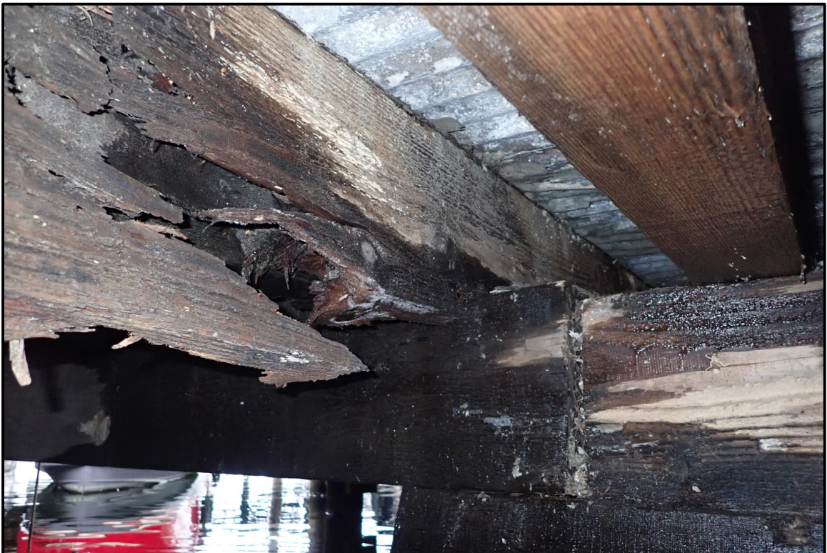
Photo 4-2: Dock C, Inshore Platform - Timber stringer crushing between the deck above and timber pile cap below due to rot.
