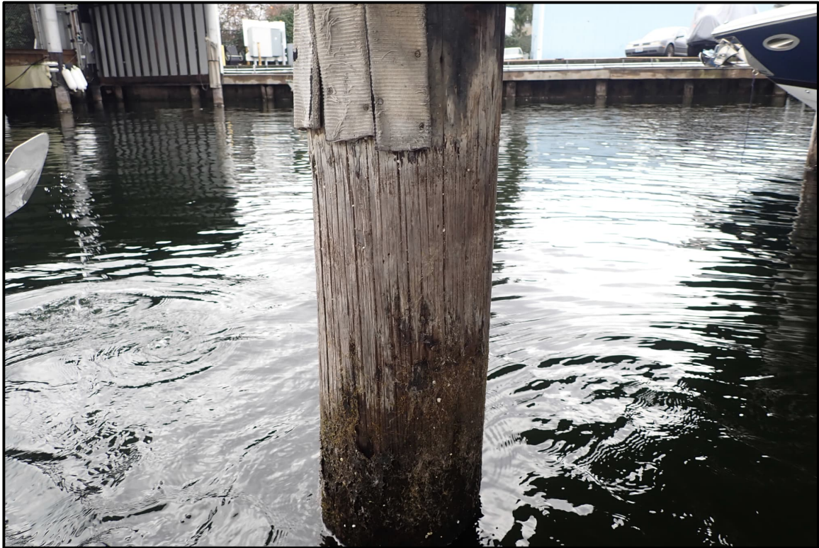
Photo 2-1: Typical timber pile ranging between 9 in. and 12 in. wide, along Docks A, B, and C.
