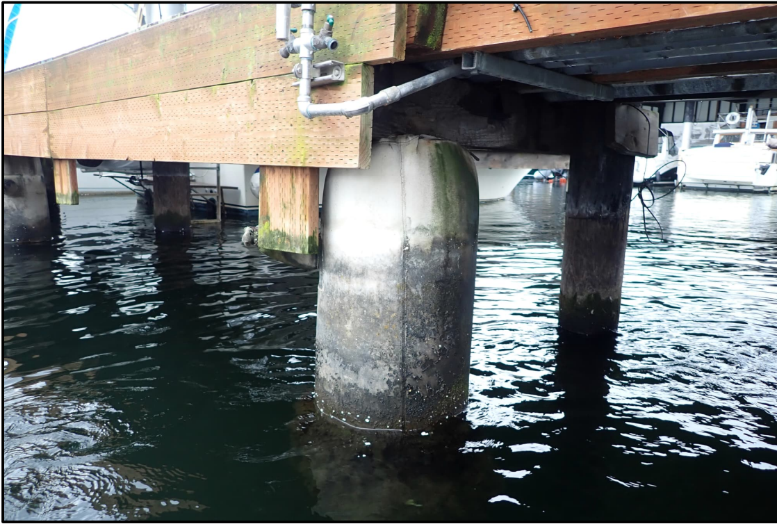
Photo 2-3: Typical concrete bag repair at Docks A, B, and C.
