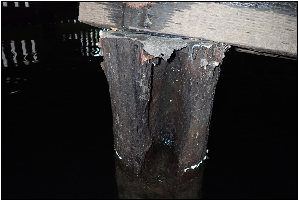
Photo 3-5: Timber pile with severe section loss due to fungal rot through core of pile.
