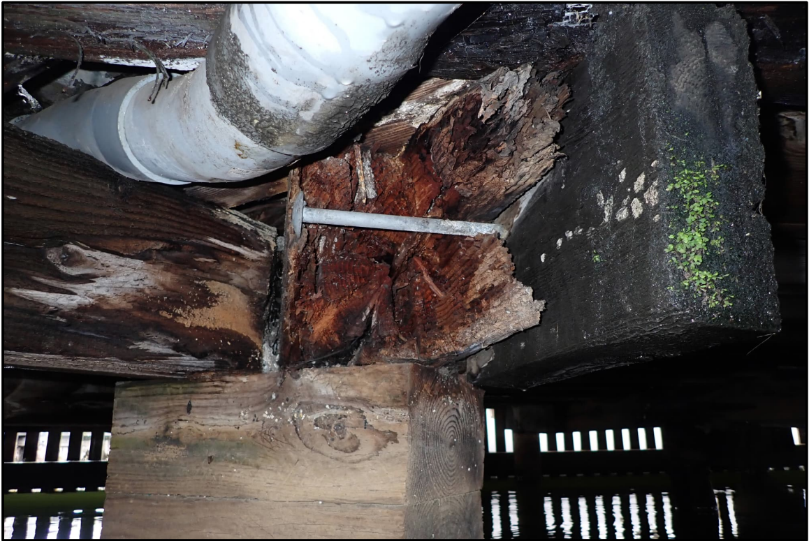
Photo 4-1: Dock C, Inshore Platform - Timber pile cap with severe section loss at its end due to rot.
