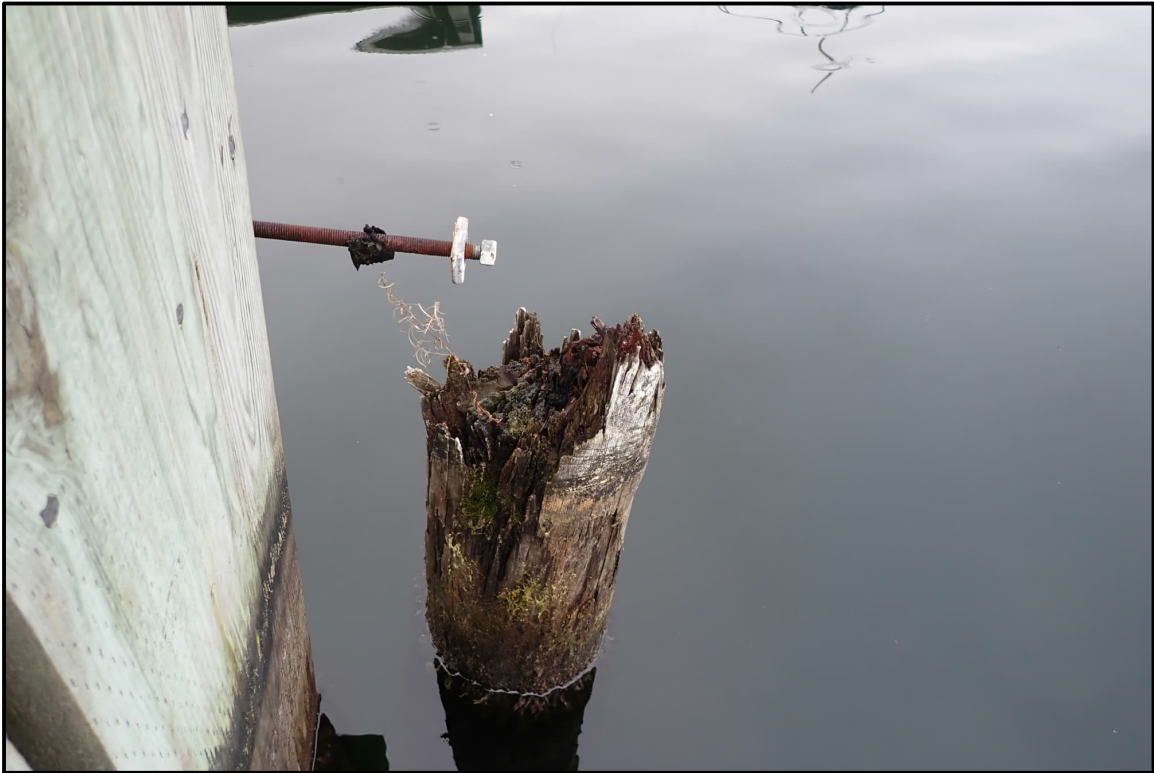
Photo 3-3: Failed connection at top of pile due to fungal rot at offshore wavescreen.
