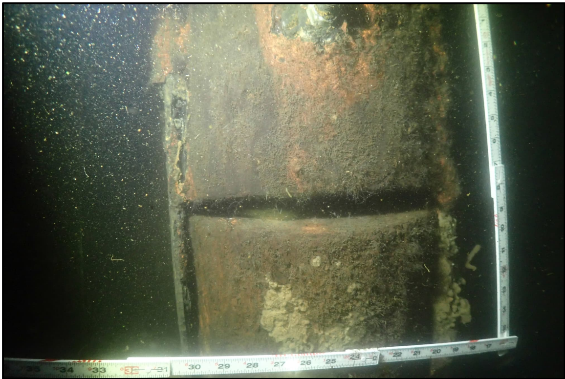
Photo 3-1: Loss of bearing at pile/post interface along the offshore wave screen.
