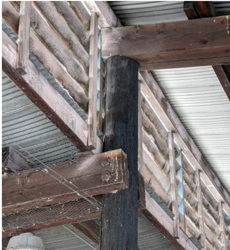
Fig 5 – Typical Girder Connections at Dock C Roof Ridge (Dock B Similar)
