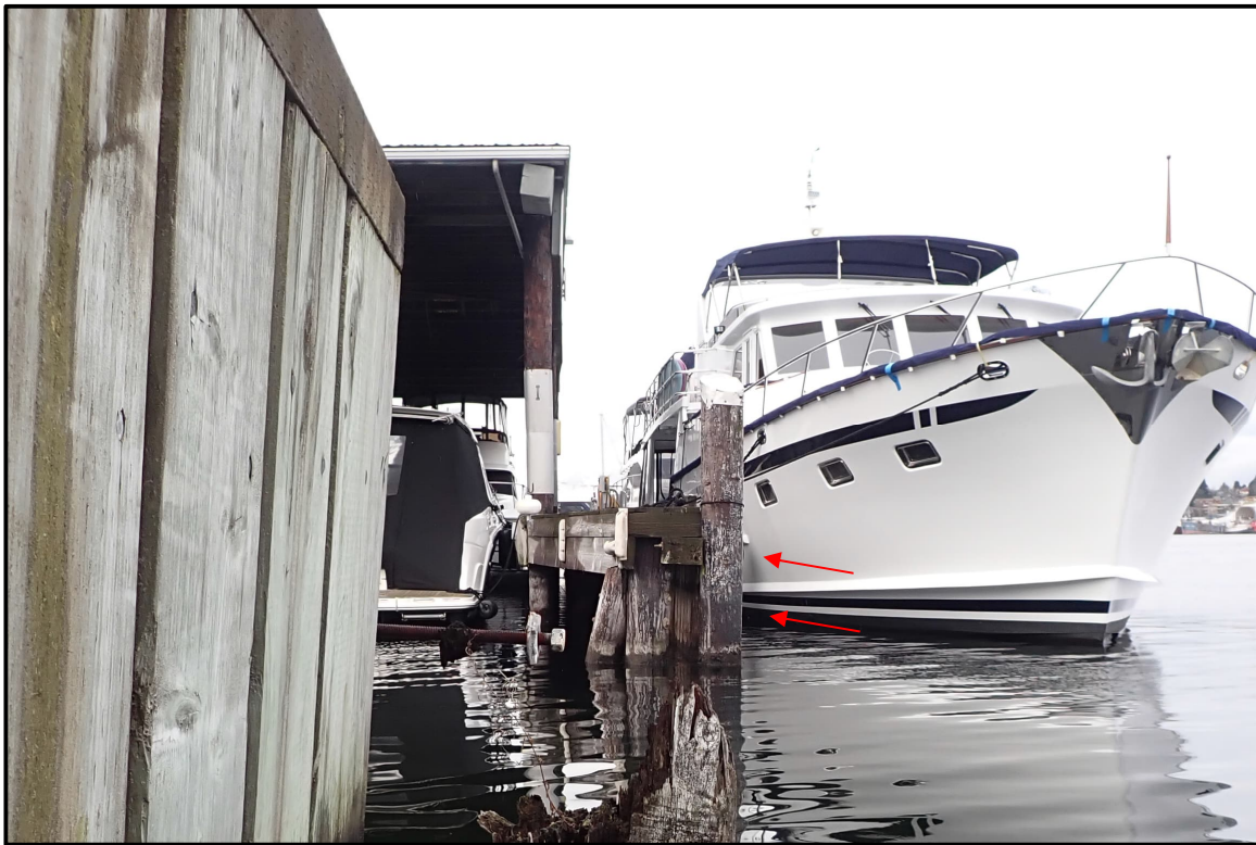
Photo 2-2: Wave screen at the offshore end of the Docks A, B and C.
