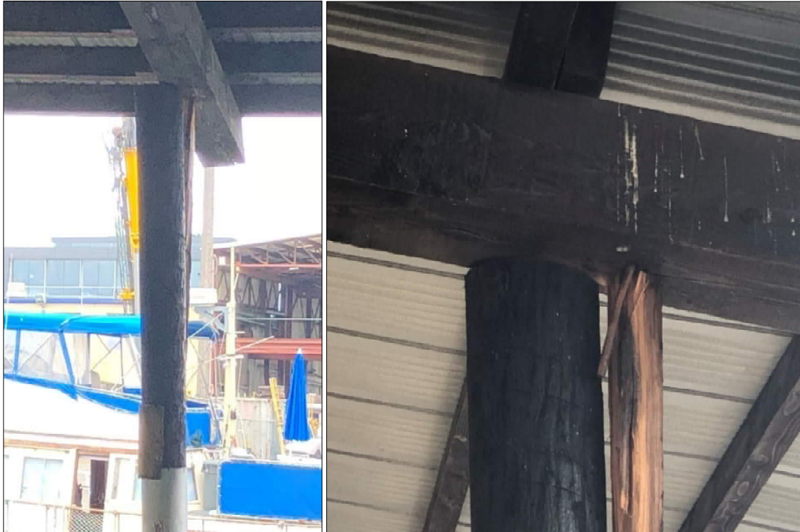
Fig 11 – 2018 Boat Impact Incident with Less Than 50% Bearing at Top of Pile and No Visible Mechanical Connection (Repaired Shortly After Incident with Channels and Thru-Bolts)
