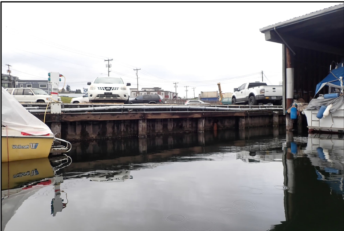
Photo 2-4: Intermittent timber piles at the face of the timber sheet pile bulkhead.
