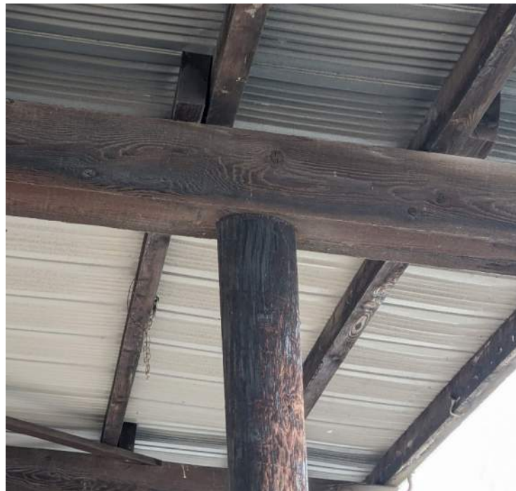
Fig 6 – Typical Girder Bearing on Pile Without Visible Connection
