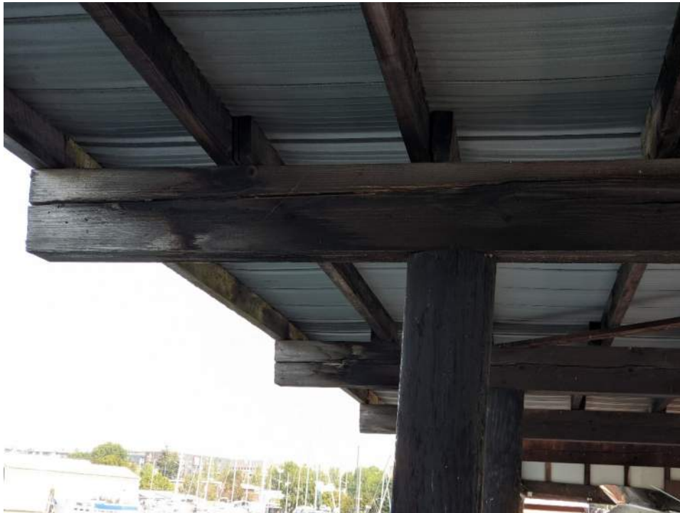
Fig 10 – Splitting and Weathering at Exposed Girder End
