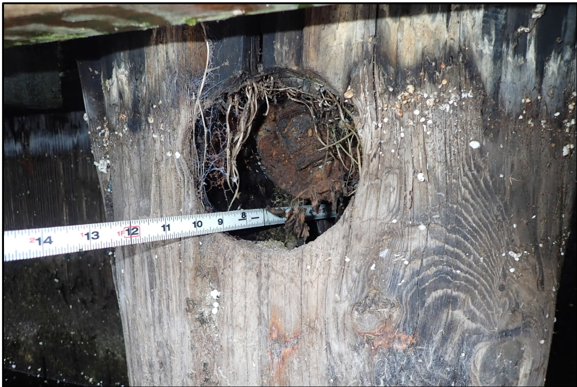
Photo 3-7: Timber pile with severe section loss due to fungal rot at top of pile along timber bulkhead.
