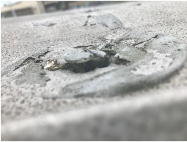
Photo 5: Fastener backout
