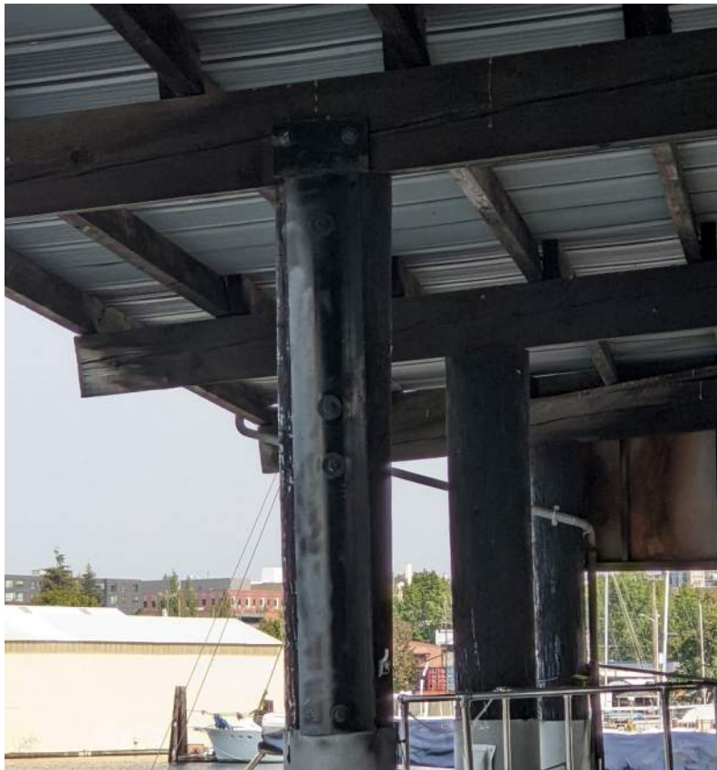
Fig 8 – Girder to Pile Retrofit
