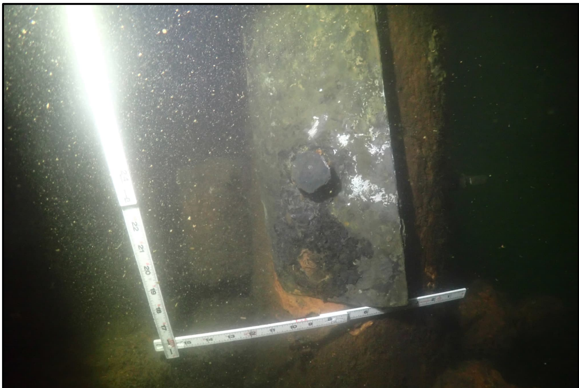
Photo 3-2: Corrosion through full thickness of steel fish plate at pile/post connection of timber pile at offshore wave screen.
