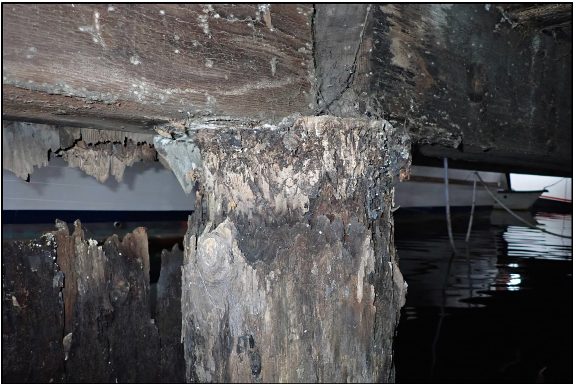
Photo 3-4: Timber pile with major section loss due to fungal rot at top of pile.
