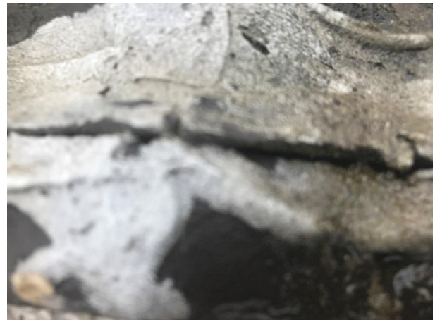
Photo 4: Failed sealant repair at seam
