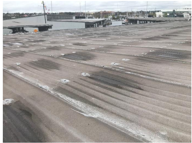
Photo 6: Ponding/Deflection between Purlins
