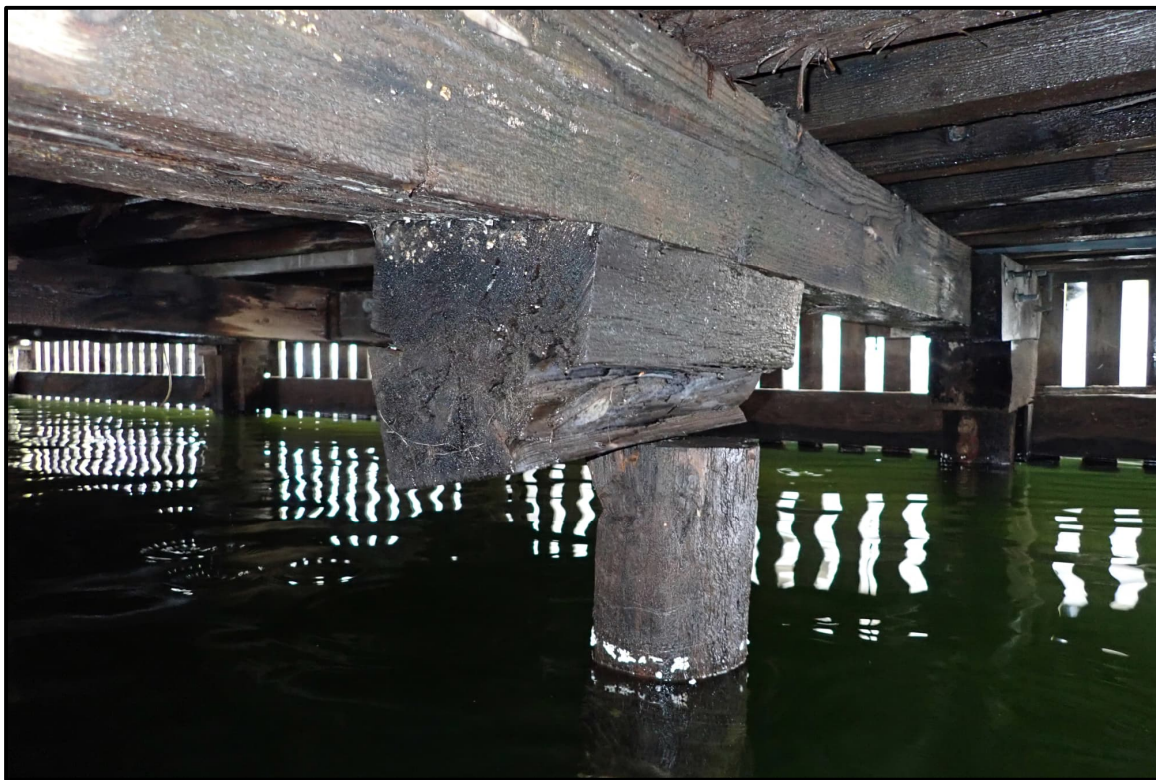
Photo 3-6: Severe reduction in bearing due to rotation and crushing of lower timber cap shimming the connection between the pile and pile cap.
