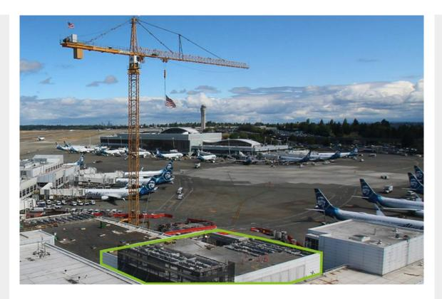
Work on the C Concourse Expansion project continues mostly behind construction walls with lots of prep work underway. The project teams have wrapped up interior demolition, waterproofed the remaining interior lower floors, and installed temporary ramp tower cameras to maintain sightlines on the airfield.
