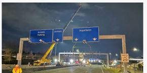
Crews successfully replaced two overhead sign bridges on the southbound Airport
