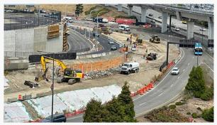
The Roadway Improvements project shifted the Departures Drive into its permanent alignment, slightly north along Air Cargo Road, earlier this summer. That created space between Departures and Arrivals drives for crews to demo and regrade the roadway in the median to prepare for two additional lanes. Coming soon, these two lanes will help alleviate congestion, provide dedicated lanes for the parking garage and courtesy vehicles, and reduce idling for private vehicles.
