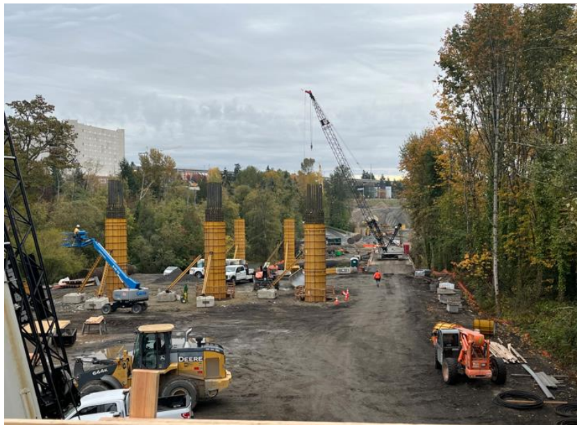
Crews build column for the future SR 509 bridge over Des Moines Creek Trail and South 200th Street
