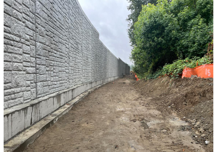
Crews placed panels for a new noise wall at South 160th Street in August
