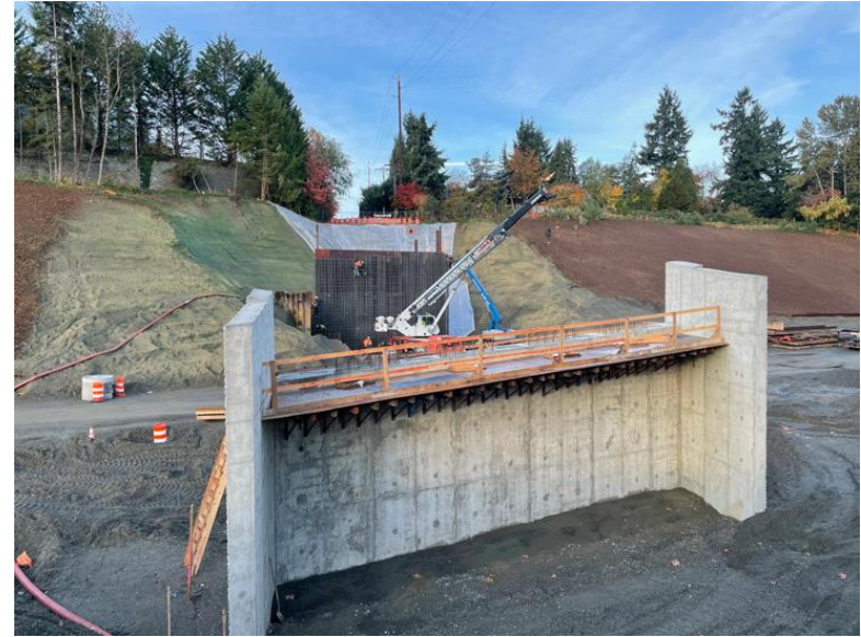
Crews build abutment walls for the new South 192nd Street bridge
