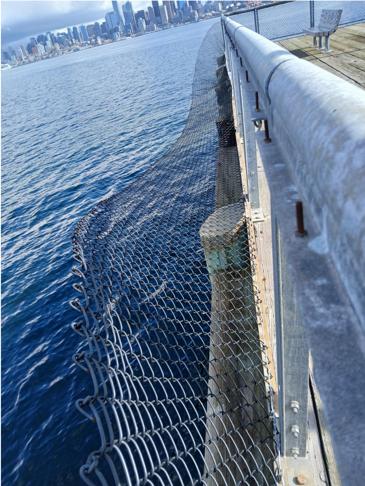
Figure 19: Jack Block Park – Pier, North Railing Separation
