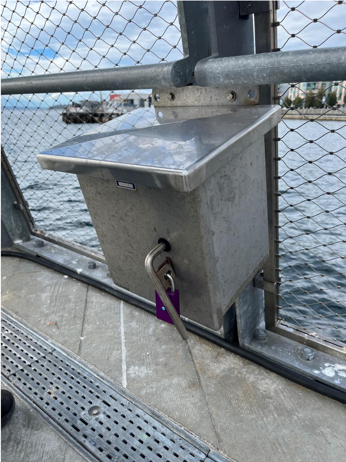
Figure 29: Pier 62 – Existing Lock Box Mounted to Railing
