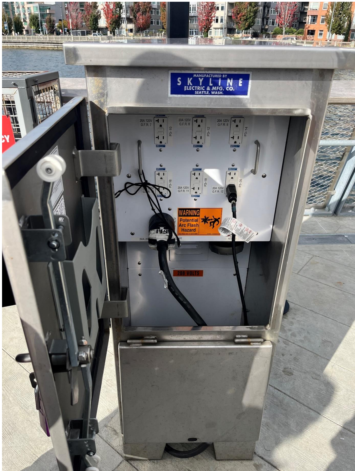
Figure 27: Pier 62 – Electrical Box with 120V 20A Power Outlets
